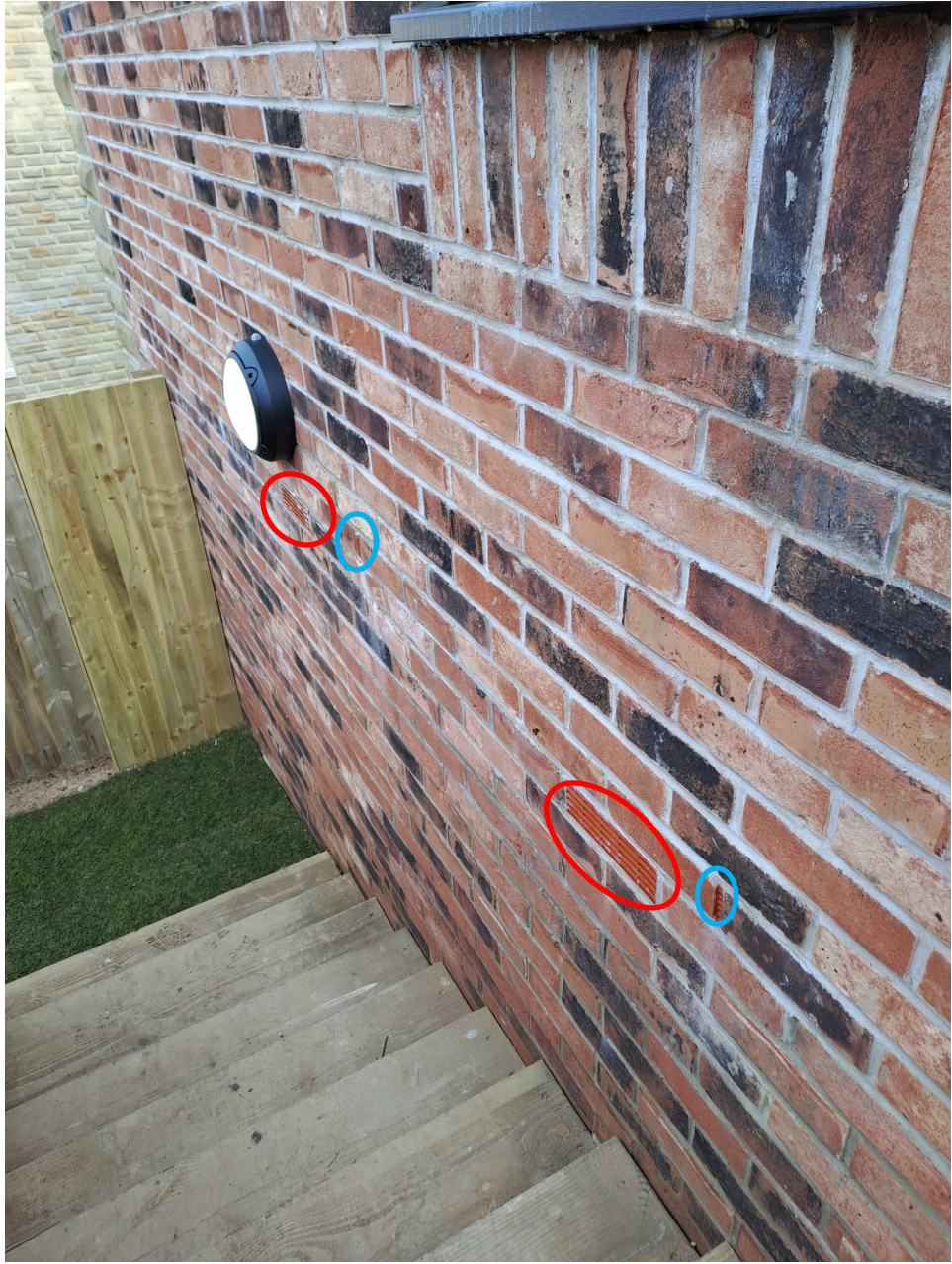
Photo 4 : Examples of vents on buildings. Air bricks (red) and weep guards (blue).
