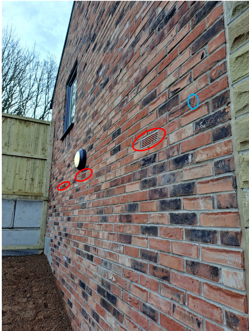
Photo 3 : Examples of vents on buildings. Air bricks (red) and weep guards (blue).
