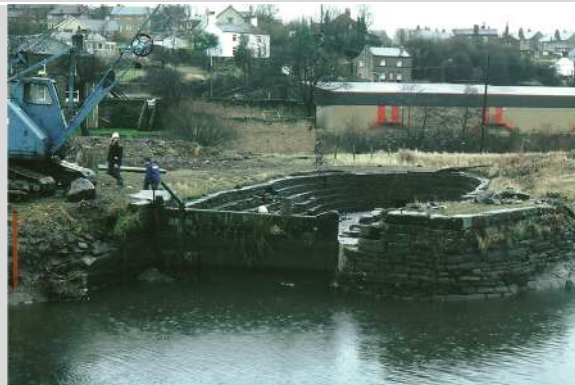
7. December 1986, excavation of new mooring basin started adjacent to the dry dock.
