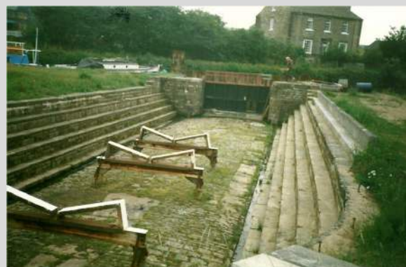
15. July 1988, new gate and boat supports installed.
