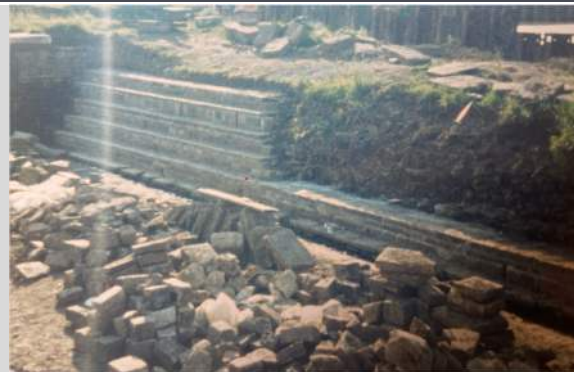
13. February 1987 rebuilding of walls with original stone.
