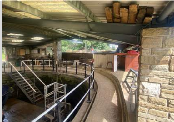
7. Northeast end of dock from inside enclosure.
