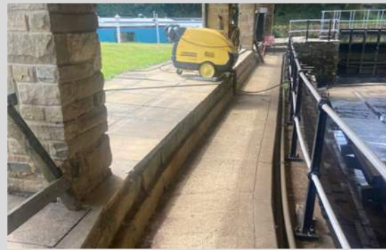
8. Southeast wall of dry dock from northeast.
