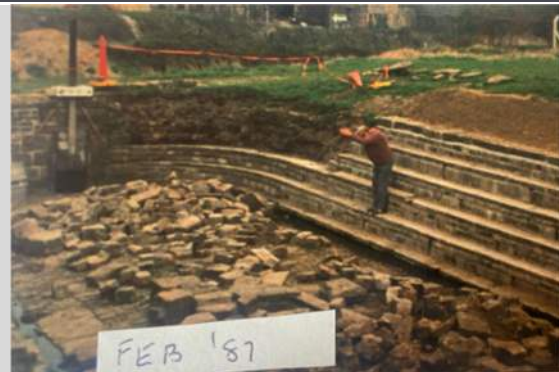
14. February 1987 rebuilding of walls with original stone.
