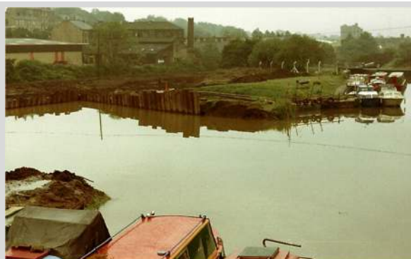
11. July 1987, basin complete
