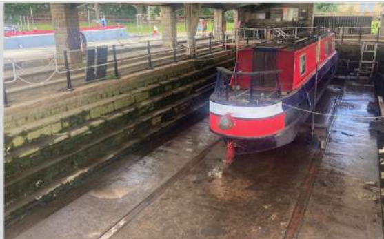
9. Dock from southeast corner of enclosure.
