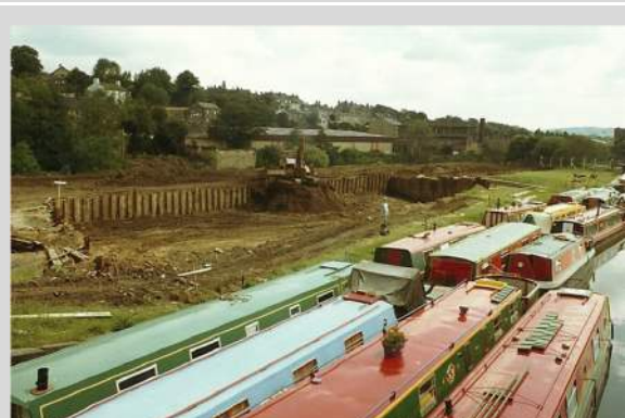
8. Basin excavations continued
