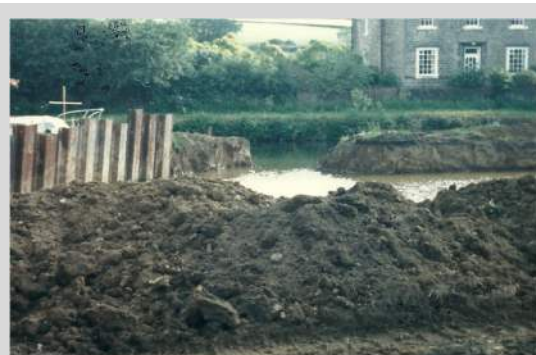
10. Arisings from basin excavation
