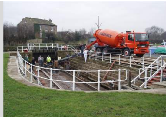
16. Reinforced concrete laid over original stonework at base of dry dock. Railings and paving slabs installed around perimeter.
