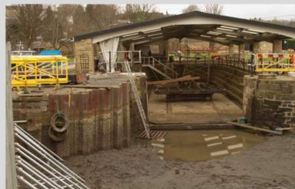
18. 2009, current day roof constructed, steel uprights clad in stone.
