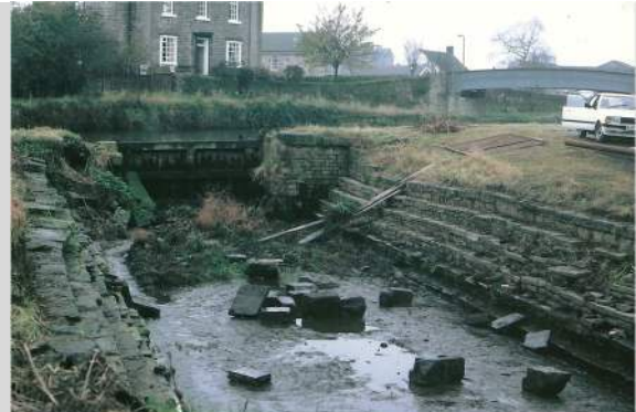
6. Spring 1986, after removal of steel bars, from northeast.
