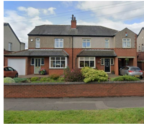
3 Semi-detached residence on Halifax Road
