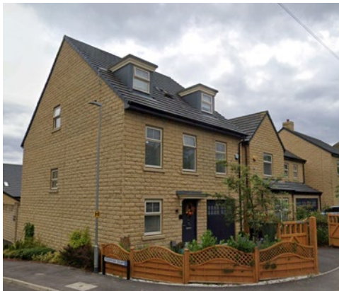
5 New build homes on New Lane
