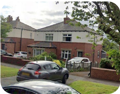
Existing house on Highmoor Lane
