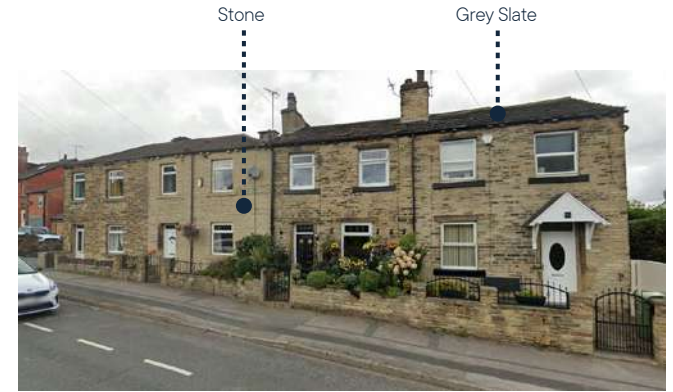
Stone terraced homes located on Moorside road, Cleckheaton
