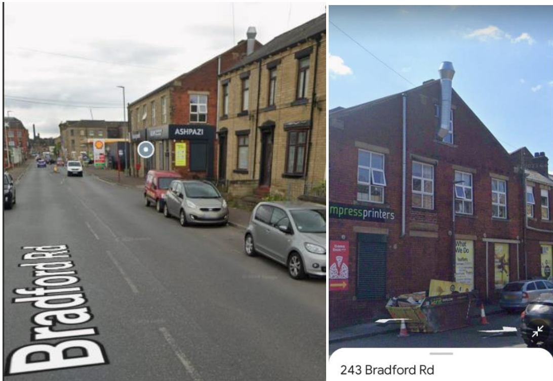
7.23 Above: Ashpazi restaurant, flue extending from window pane in a prominent position.
