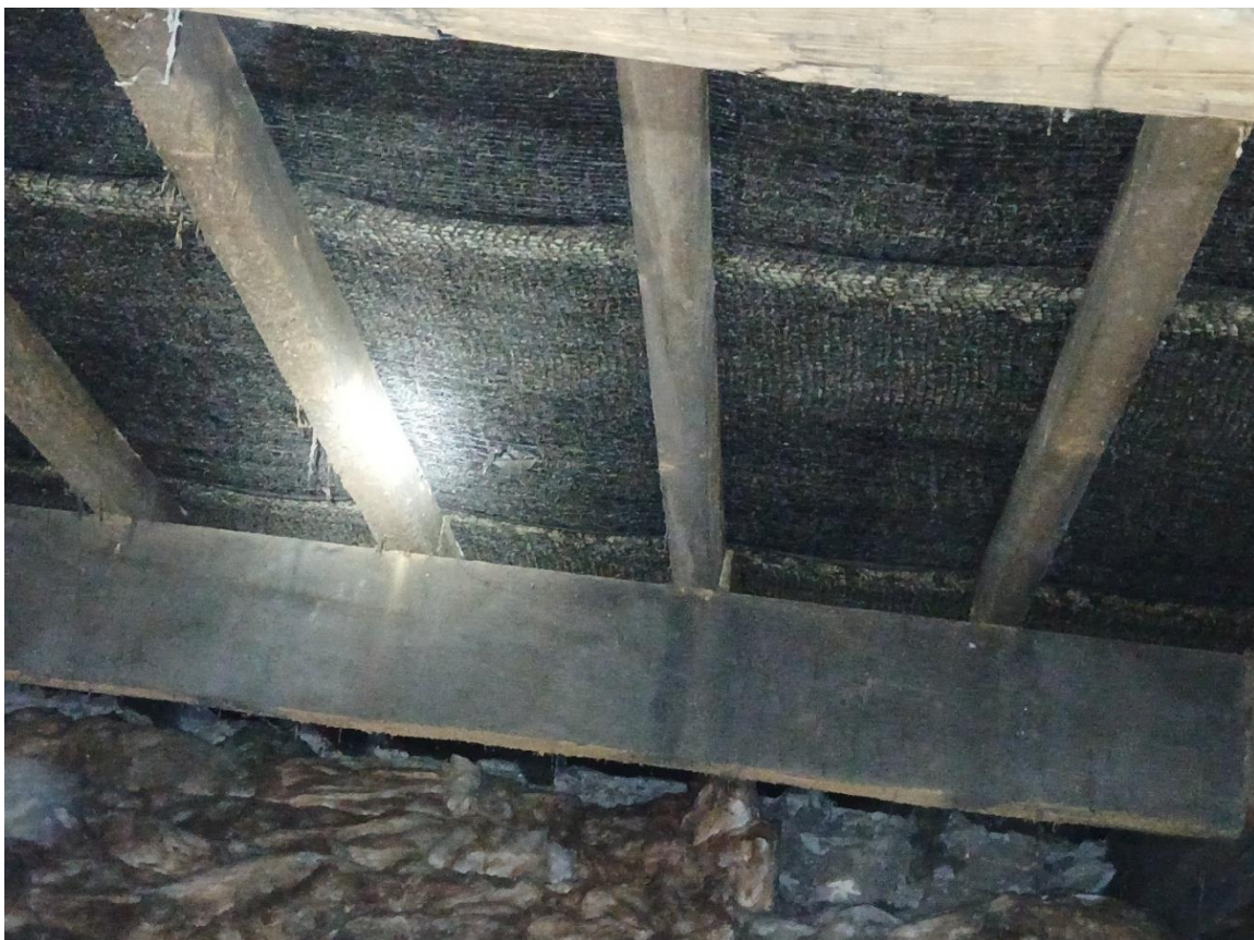
Photo 26: Southwest side of the loft, gap in the upper insulation with light coming out.
