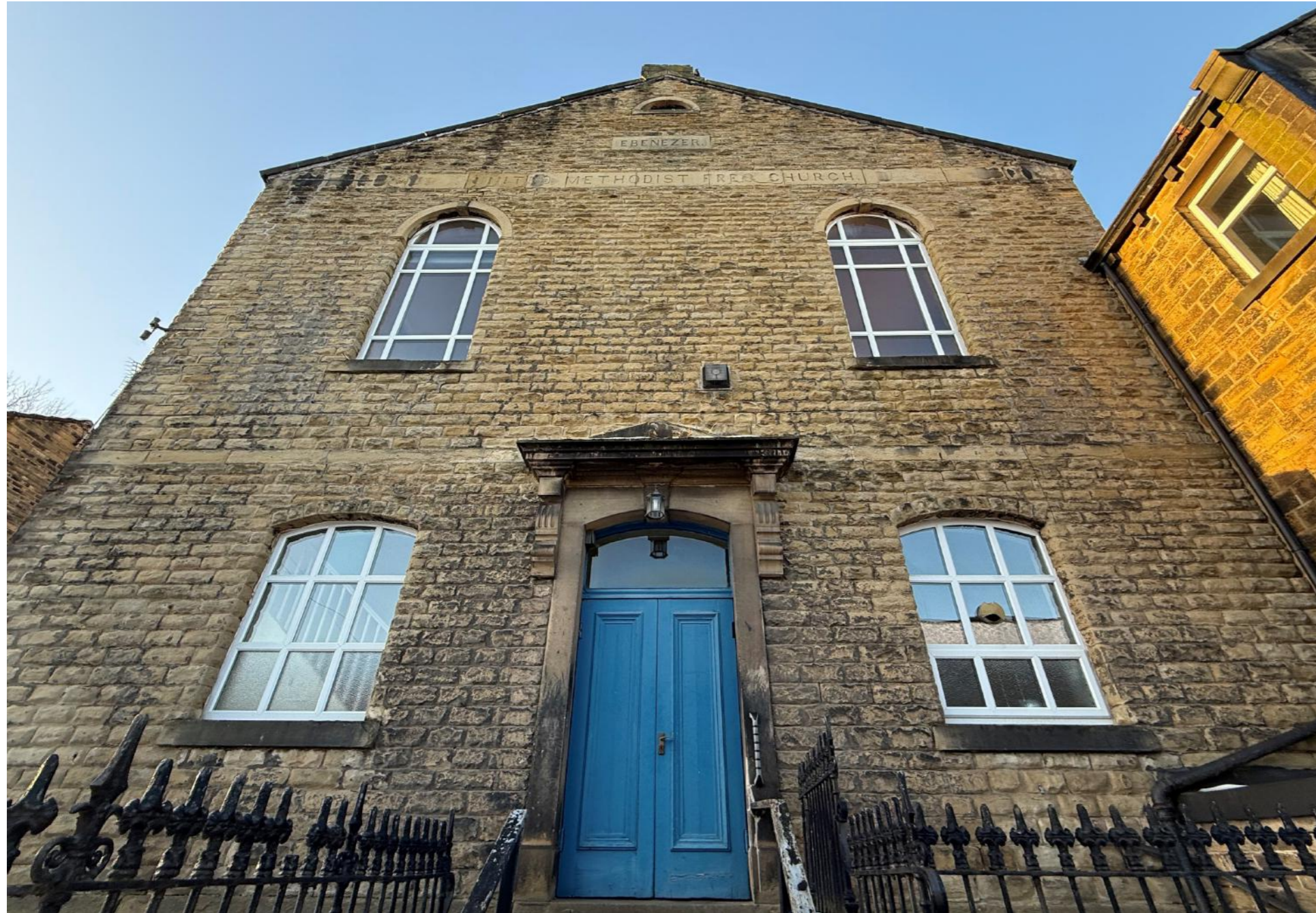
Existing main entrance
