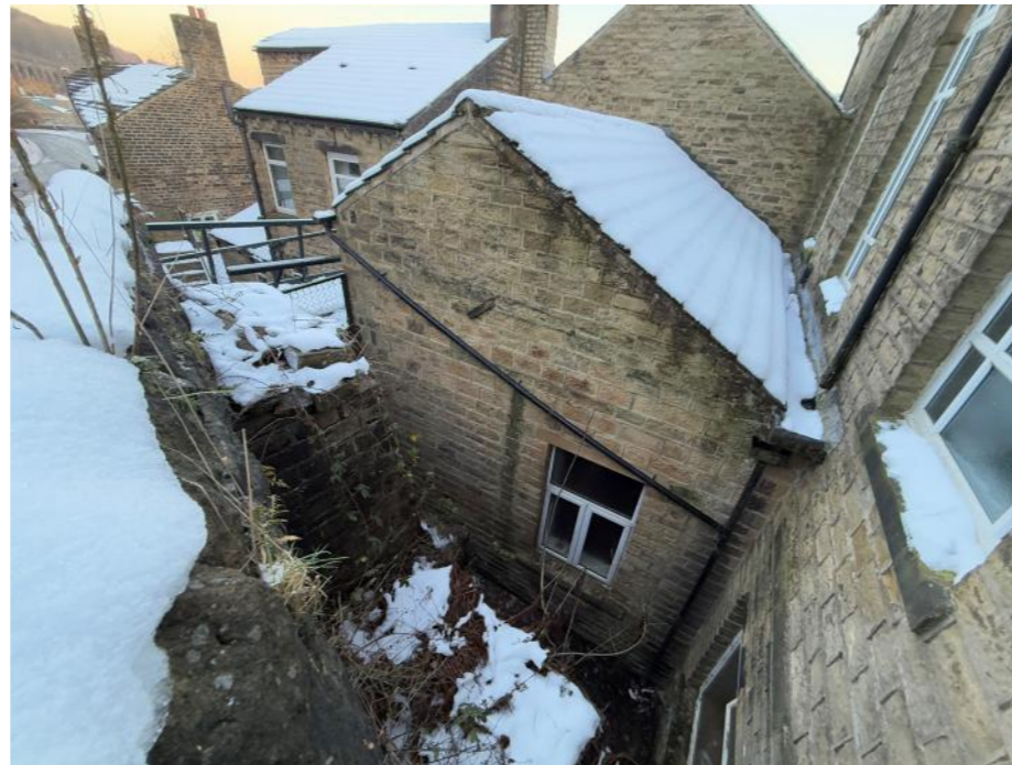
5. View looking into the existing lightwell from Station Road
