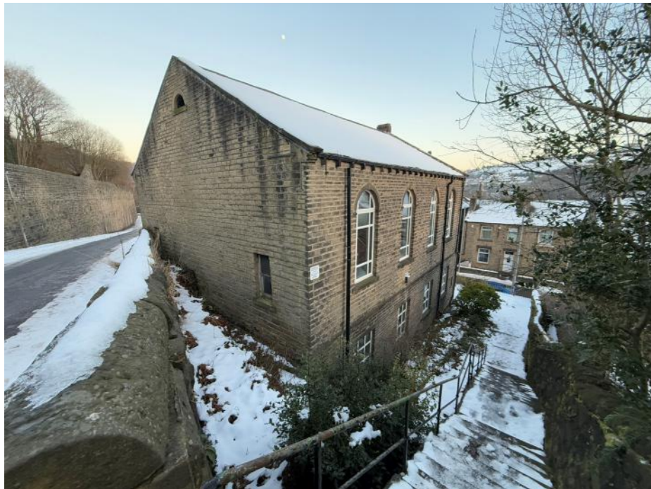
4. View looking down the site from Station Road
