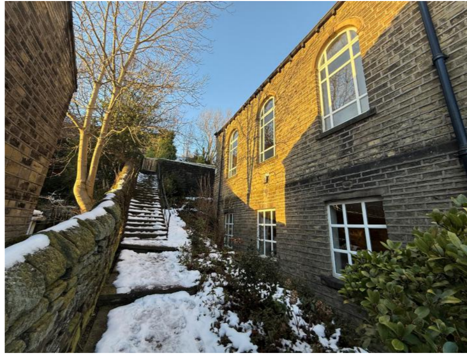
2. View up side of site to Station Road
