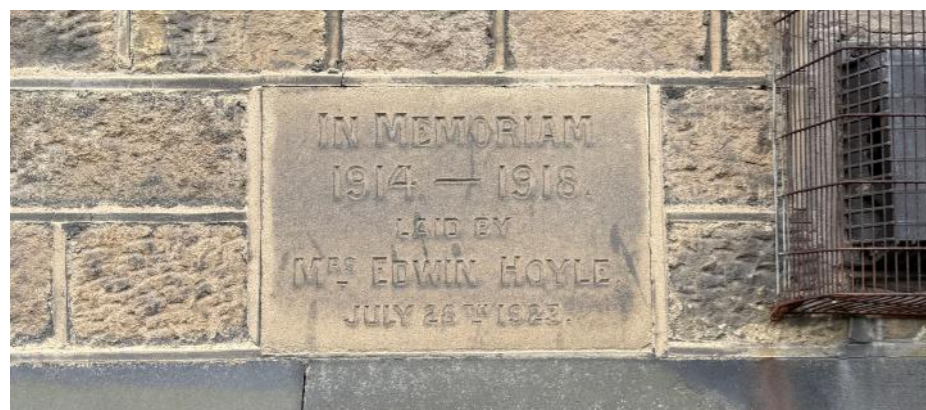
Existing memorial stones on the front of the Sunday School extension
