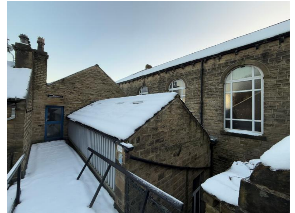
6. View towards the first floor entrance from Station Road
