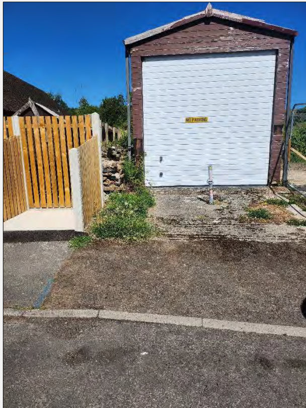
Plate 1: Small garage unit to southwest of site north of Olney Street
