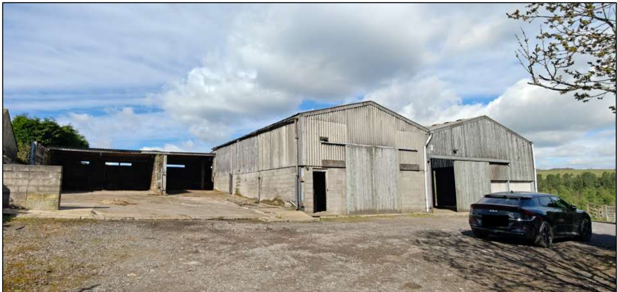
Agricultural Buildings (east elevation) – Holt Farm
