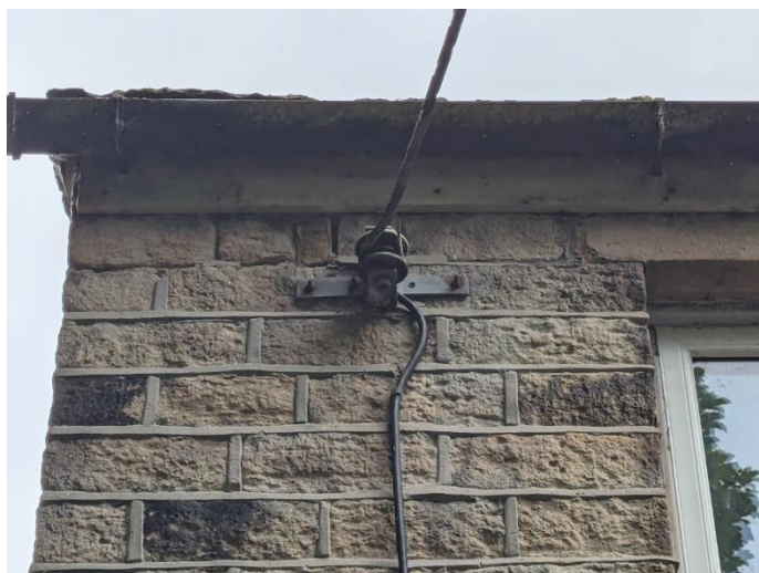
Figure 25 Gap to mortar - north elevation
