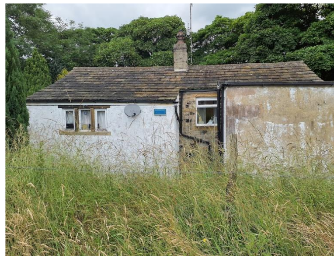
Figure 24 View of southern roof pitch
