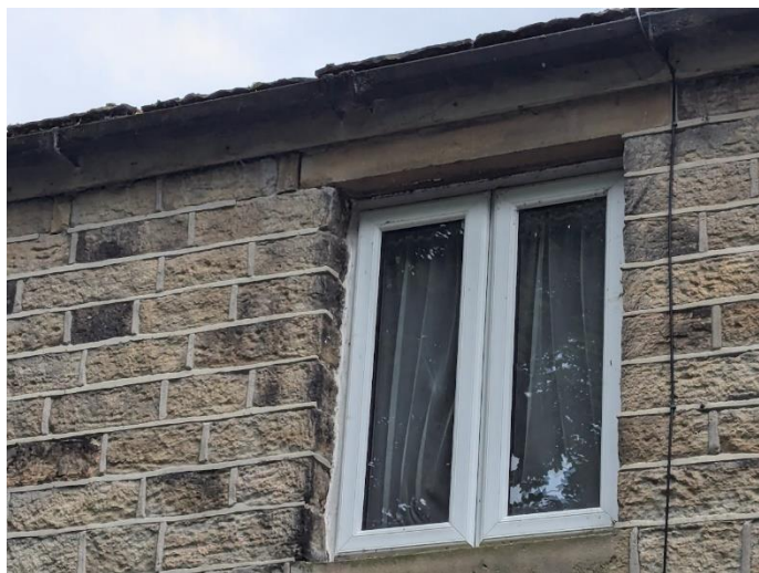
Figure 25 Gap to mortar - north elevation
