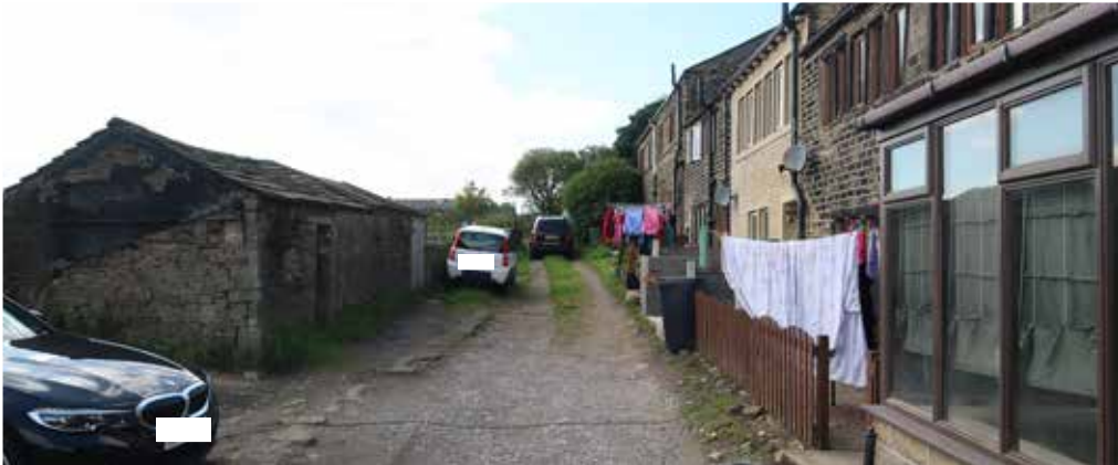
Image top: Showing the possible change in articulation of the buildings which may represent a first and second phase of construction. Centre: The juxtaposition between the end barn element and the cart house. Bottom: Similar buildings nearby where the single storey ancillary building still survives. At Round Ings there would appear to have been such a building immediately opposite the main range but this seems to have been ruinous by the 1970’s.
