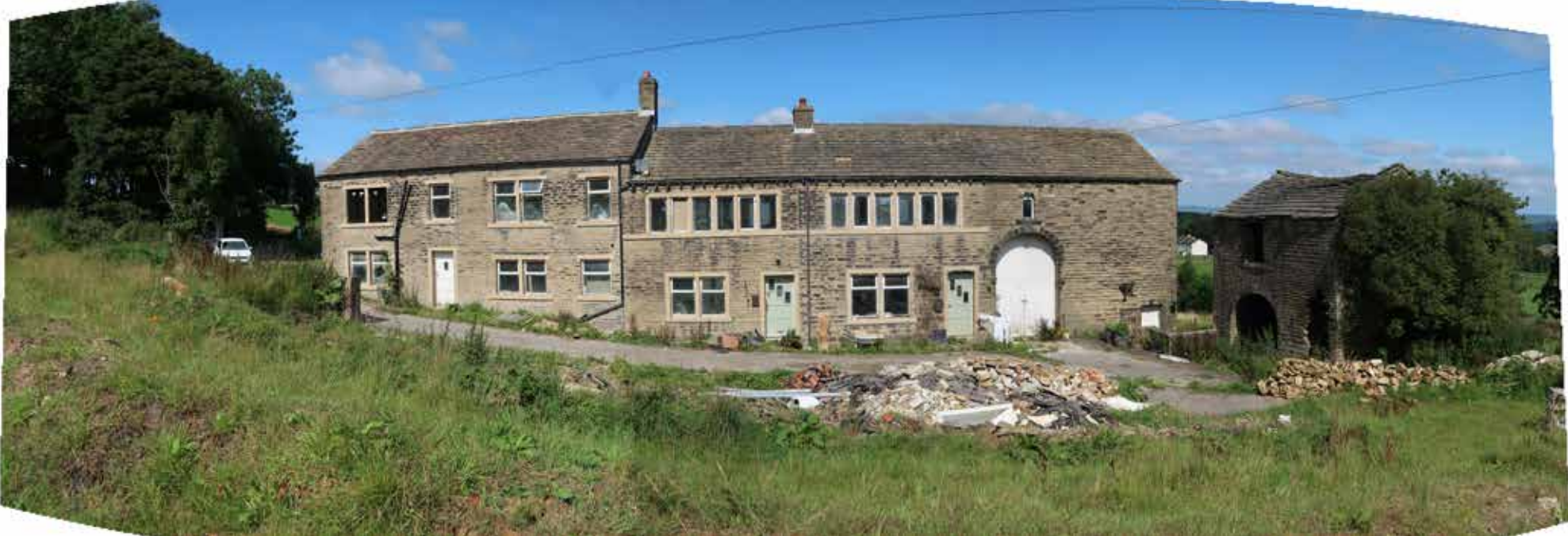
Image Below: Panoramic image of the south facing (front) elevation of the building showing the changes in character from detached cart shed to barn, to workers range and perhaps the owner's house to the left hand side.
