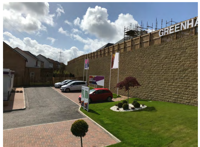
6m retaining wall height on housing development
