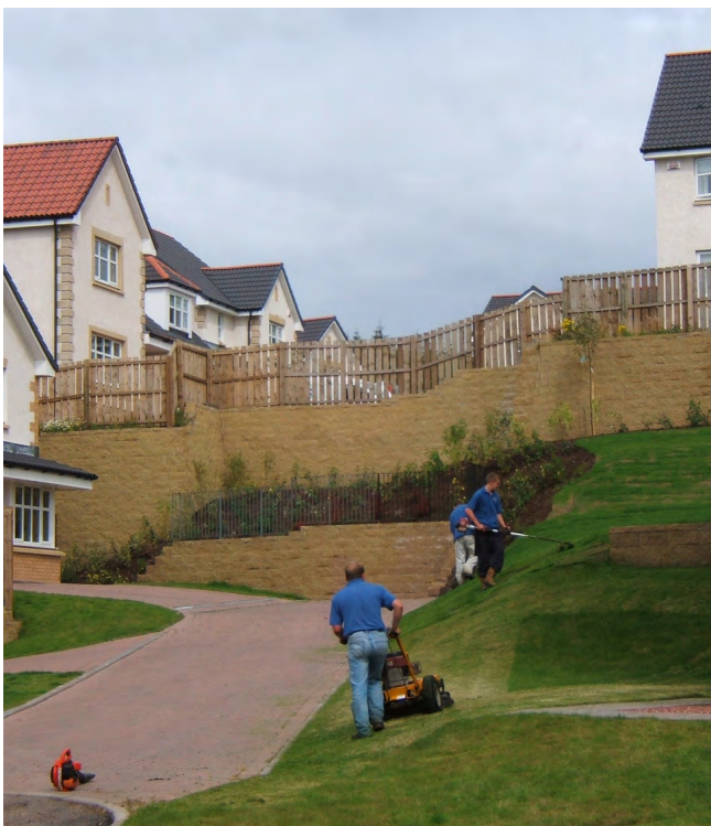
Corners and curves are simple to build
