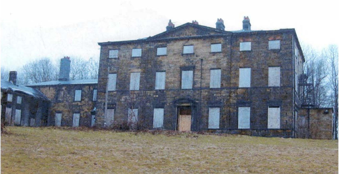
Archive photo of the south elevation of The Mansion House at Storthes Hall (pre 2000). Roof sheeted and windows blocked. Fire escape in place to the east elevation, along with extension.
