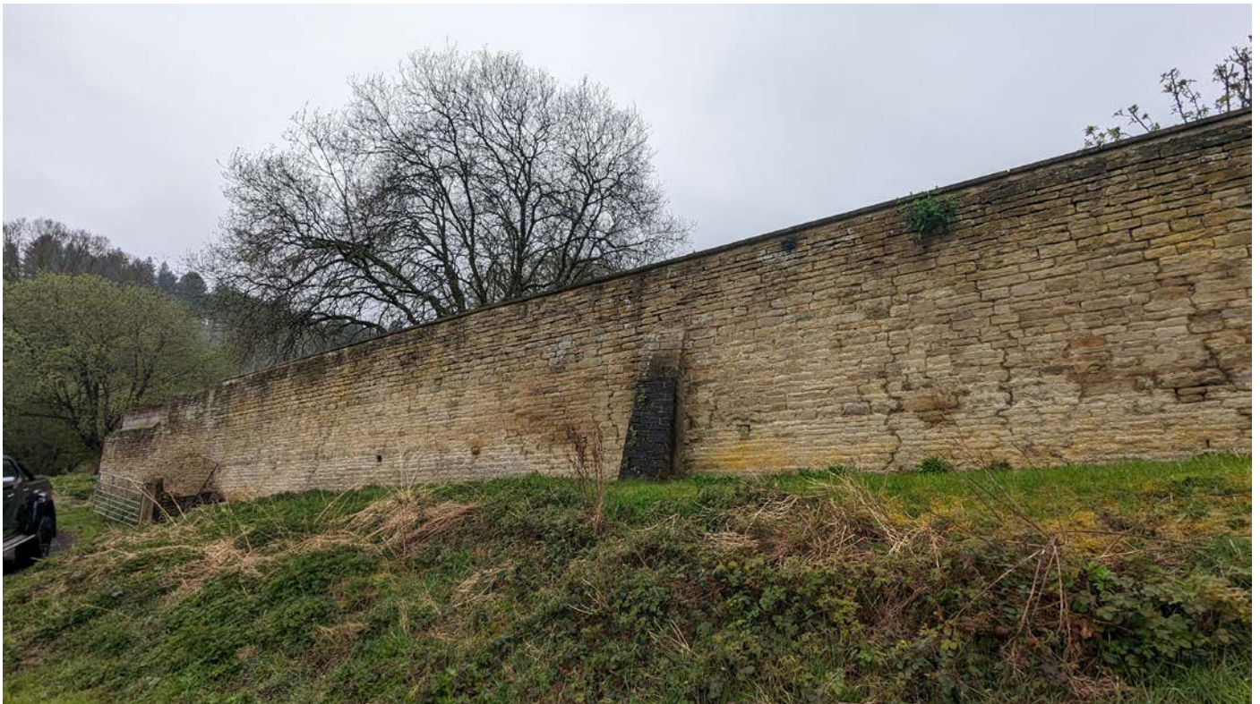
Walled garden, path to store. Top of breezeblock visible to the left of the image. Copings are modern (concrete). (Author, 2024)
