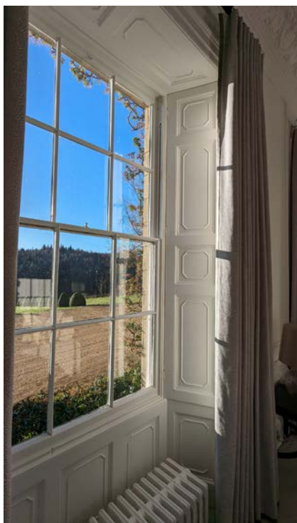
Ground Floor Window (Author, 2024) Historic timber windows and cast iron radiators repaired
