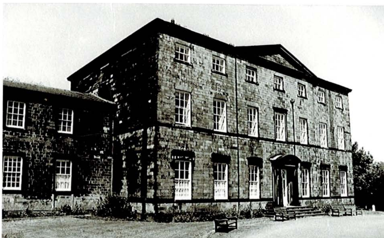
Archive photo of the south elevation of The Mansion House at Storthes Hall, Huddersfield (circa 1986).
