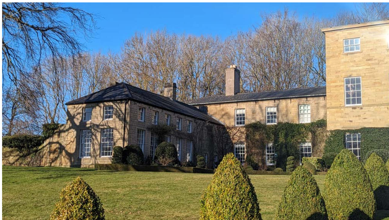
South Elevation of West Wing (Author, 2024) Top left hand window converted from blocked opening to window circa 2001
