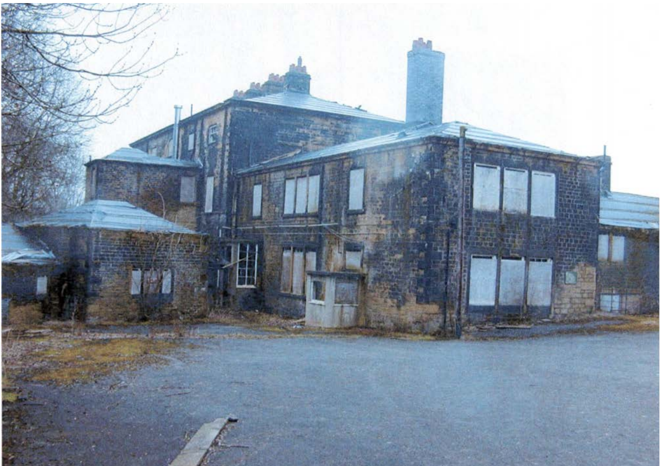
Archive photo of the west elevation of The Mansion House at Storthes Hall (pre 2000). This shows the car park and two porches to the north entrance of the West Wing.
