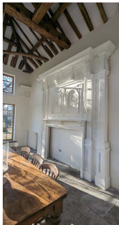
Orangery (Author, 2024) Plaster ceiling lost, reclaimed fire surround introduced
