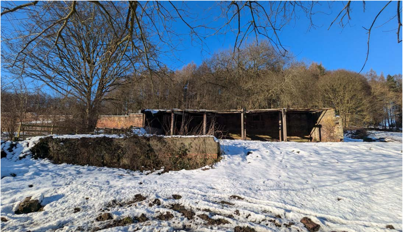
South Elevation of existing store - the existing store detracts from the setting due to its poor condition.
