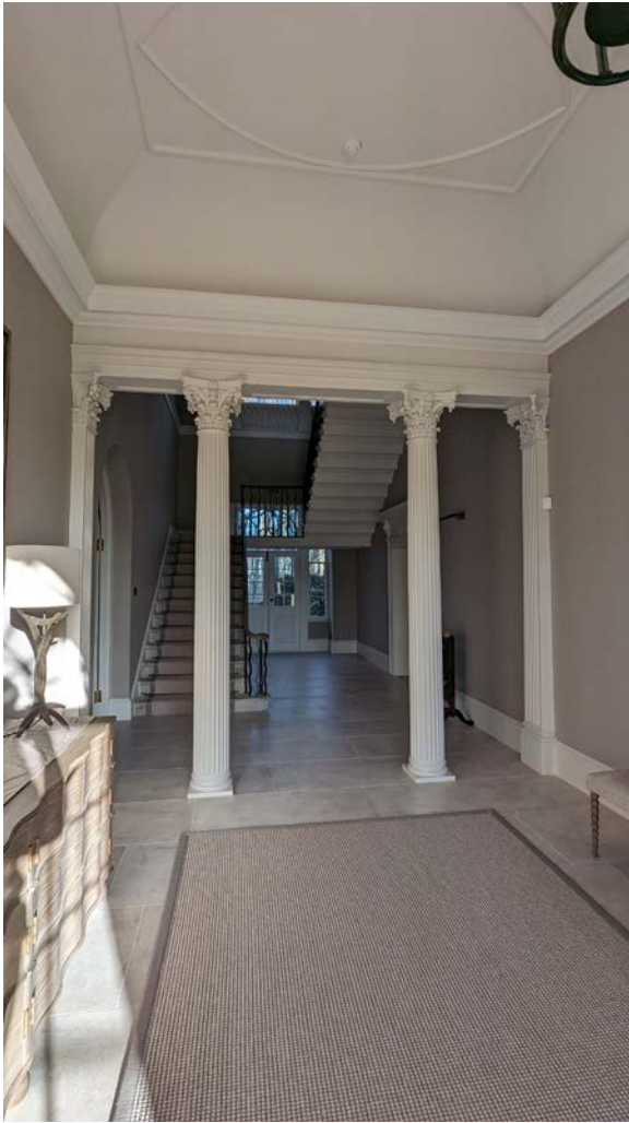
Entrance - columns (modern replacement to match existing), historic cantilever stair and ironwork (Author, 2024)
