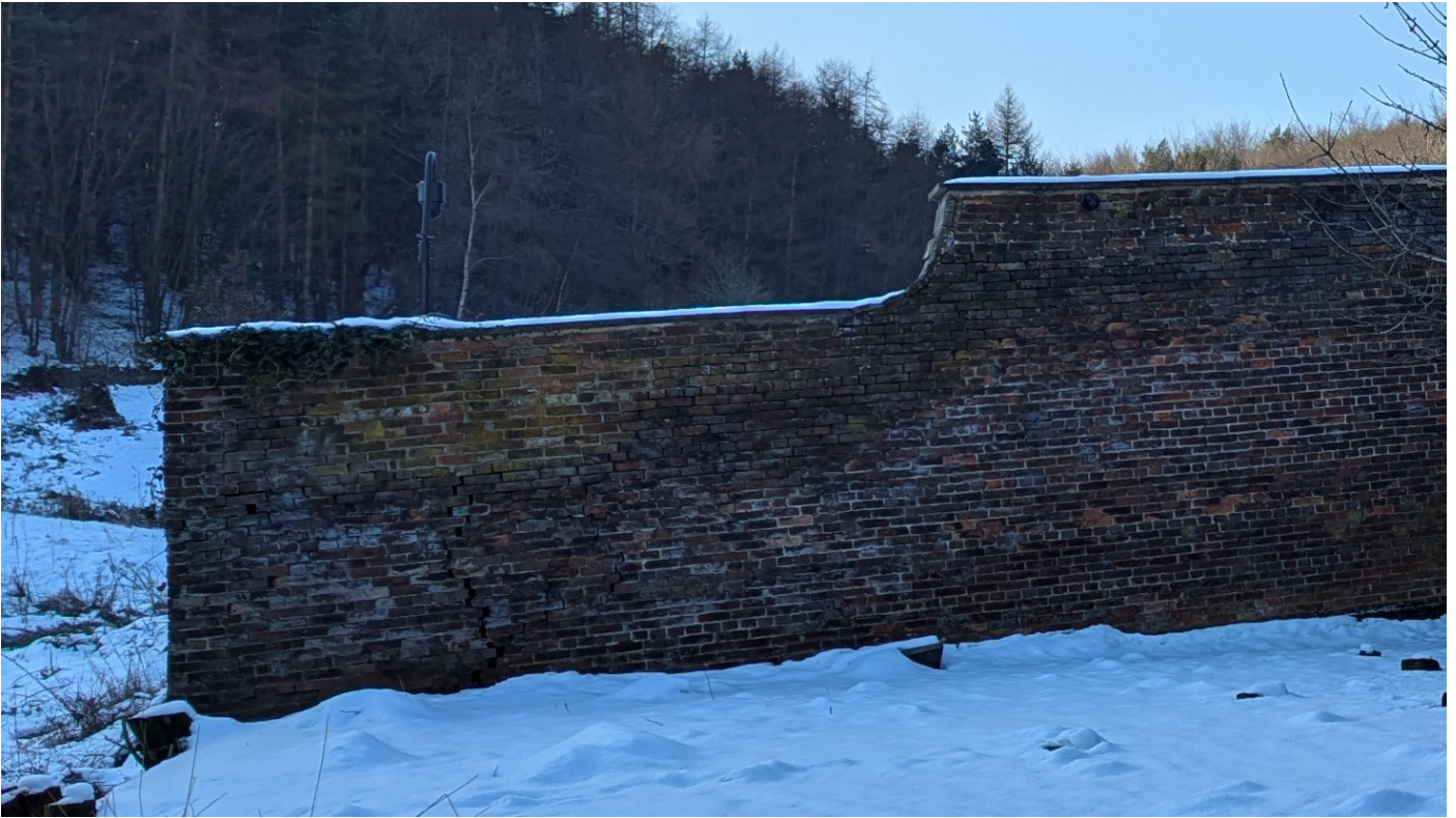
Existing wall to the west with curved feature intact - to be replicated in the proposal.
