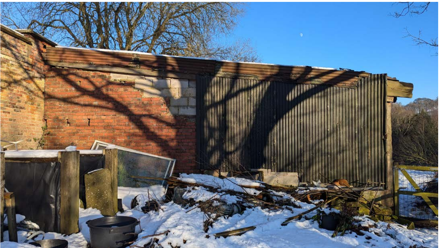
Existing store, west elevation showing corrugated sheeting, breezeblock and modern brick construction.
