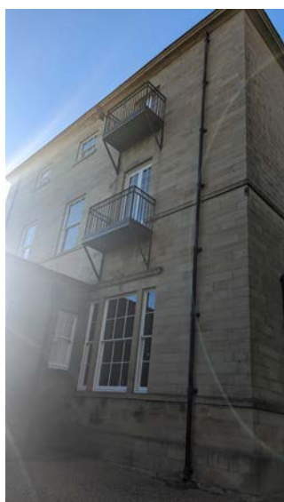
East Elevation (Author, 2024) Fire escape removed and balconies fitted circa 2001
