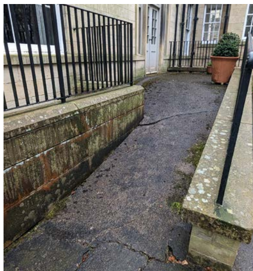
Concrete ramp (Author, 2024)
