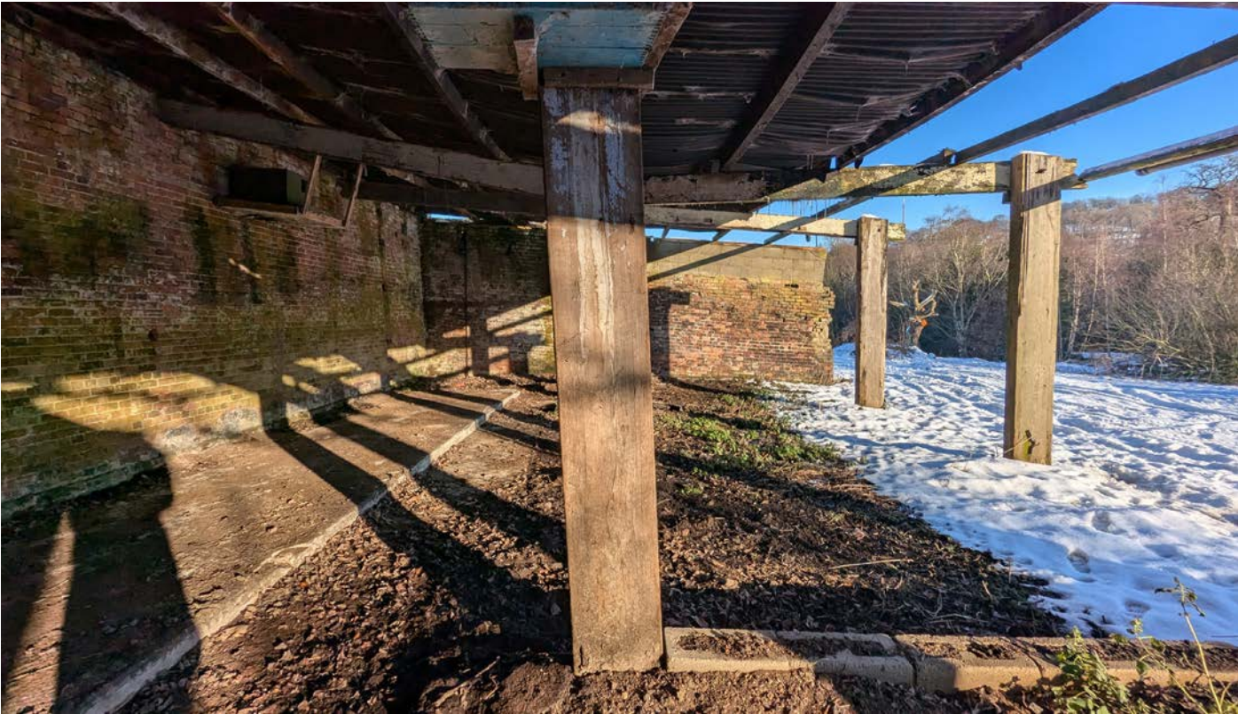
Existing store, looking east, showing existing concrete slab, timber framing and breezeblock construction.
