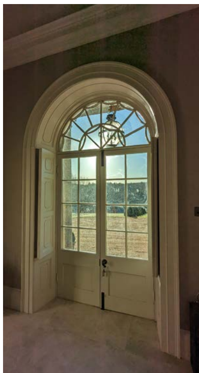
Entrance Door (Author, 2024) Historic timber doors with modern glass replacements
