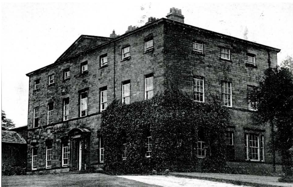
Archive photo of the south east of The Mansion House at Storthes Hall prior to extension.
