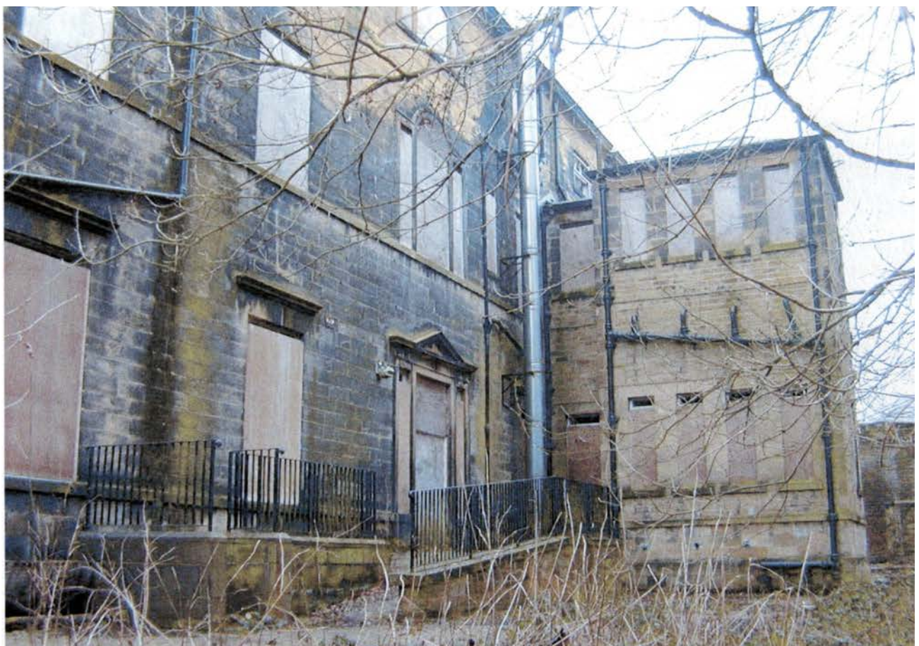
Archive photo of the north elevation of The Mansion House at Storthes Hall (pre 2000). This shows the extension and ramped access added circa 1925.
