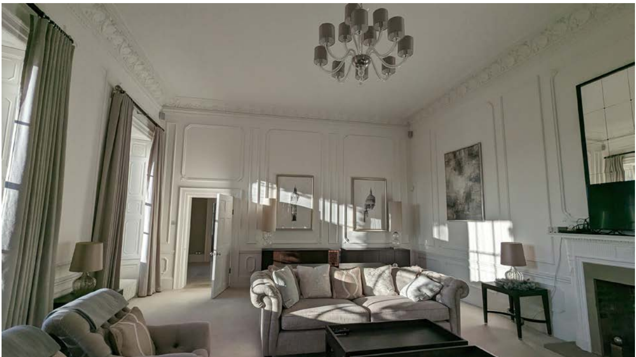
Drawing Room - plasterwork, modern to match existing (Author, 2024)
