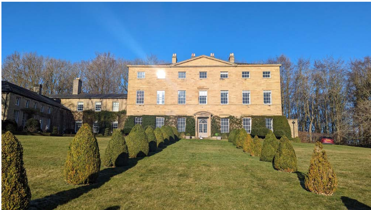
South Elevation of Mansion House (Author, 2024) Stone cleaned circa 2001
