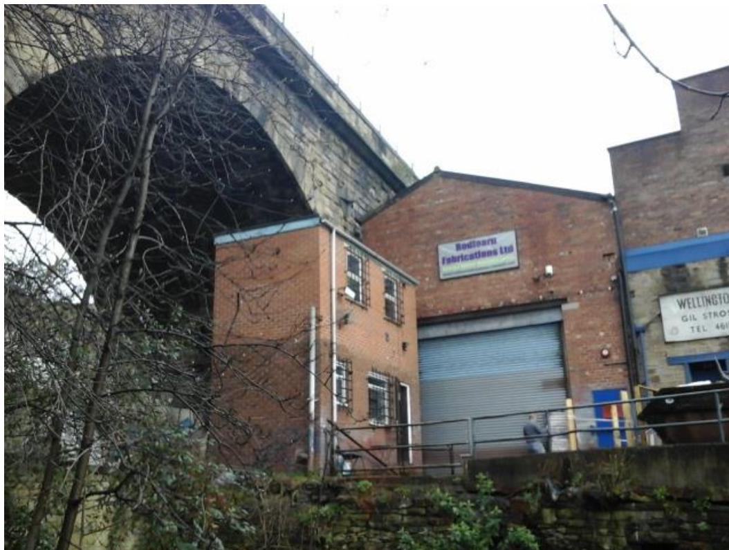
Insert 2-8 Span 8 showing abutting buildings (eastern elevation).
