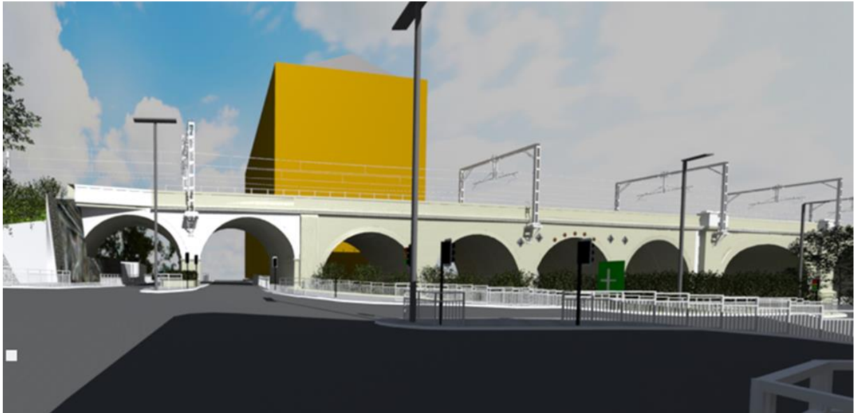
Insert 3-2 Indicative visualisation showing the OLE portals along the viaduct. Note the position of this visualisation is represented by viewpoint 3 indicated by the map in Insert 3-1 above.
