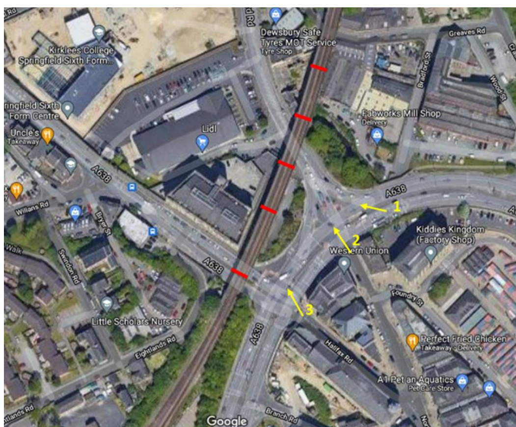
Insert 3-1 Aerial view showing locations of OLE portals (represented by the red lines across the structure). The yellow numbers and arrows indicate the locations of viewpoints from the edge of the Dewsbury Town Centre Conservation Area (see Insert 3-2 below).
