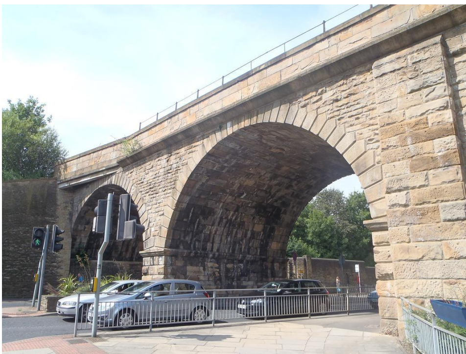
Insert 2-2 Spans 1 and 2 over Halifax Road (eastern elevation).
