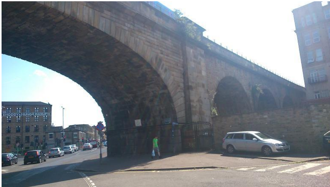
Insert 2-5 Projected pilaster, Span 7 (western elevation).
