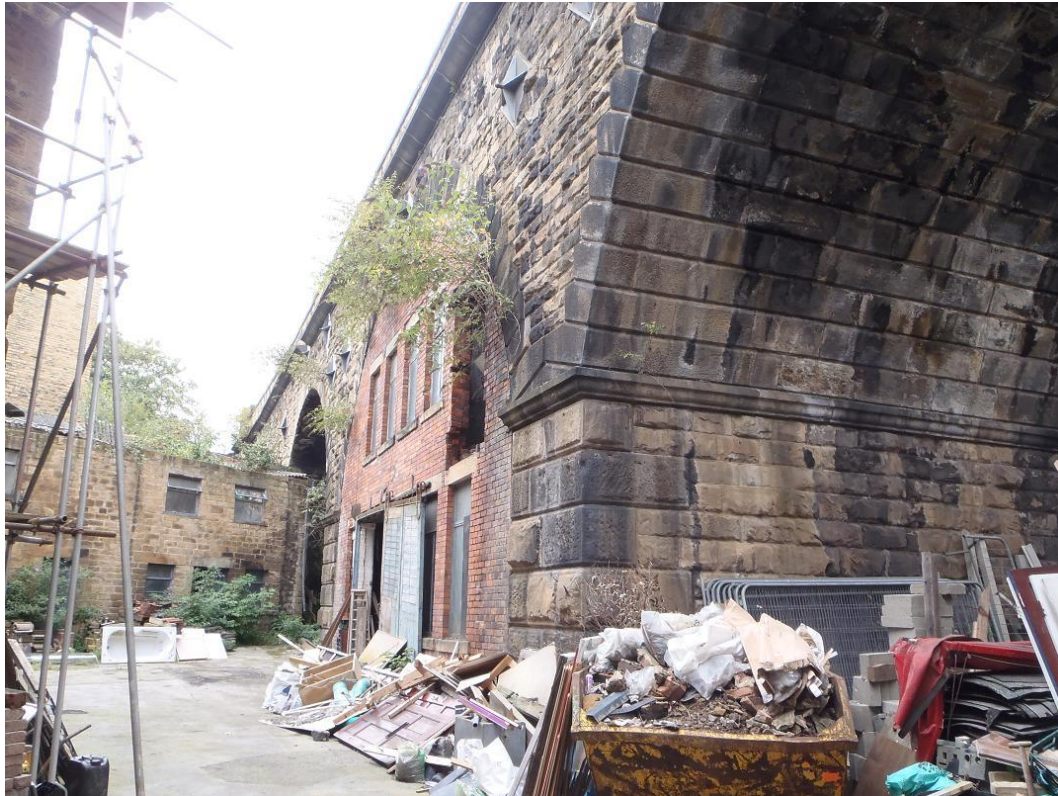
Insert 2-6 Spans 8,9 (with red brick infill) and 10 (western elevation).
