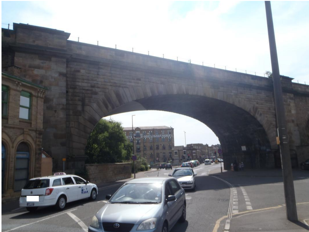
Insert 2-3 Span 7 over Bradford Road (western elevation).
