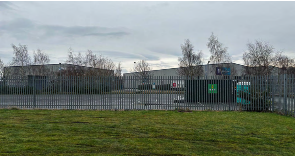
3 - Picture 3 View looking towards car park
