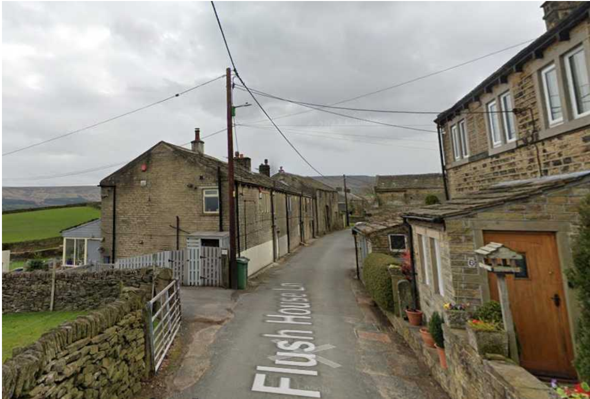
Figure 3: View of the east elevation of the listed building on approach along Flush House Lane
