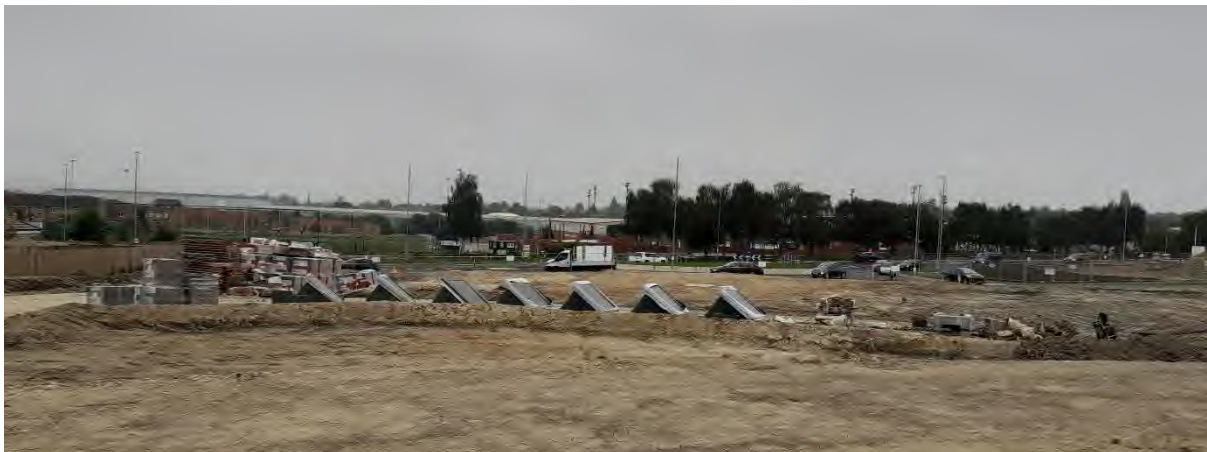
Photograph 07: Material laydown area in the southwest of the Phase 2 site (18.08.23).
