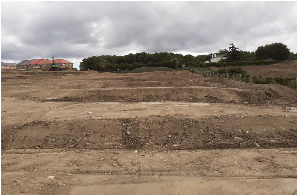
Photograph 13: Looking northeast over the finished site (07.08.23).
