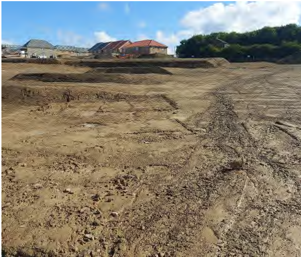
Photograph 11: Plot layout looking north-northeast (03.08.23).
