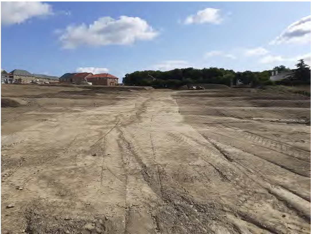
Photograph 15: Site development at finished remediated level (08.08.23).
