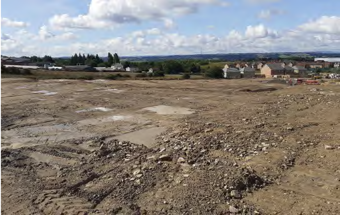
Photograph 12: Looking southwest over the finished site (03.08.23).
