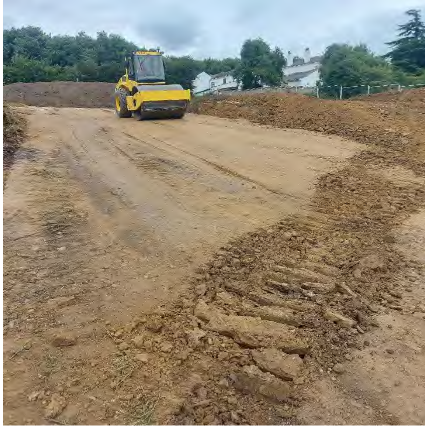
Photograph 03: Cut and fill operations with compaction of engineered fill (18.07.23).
