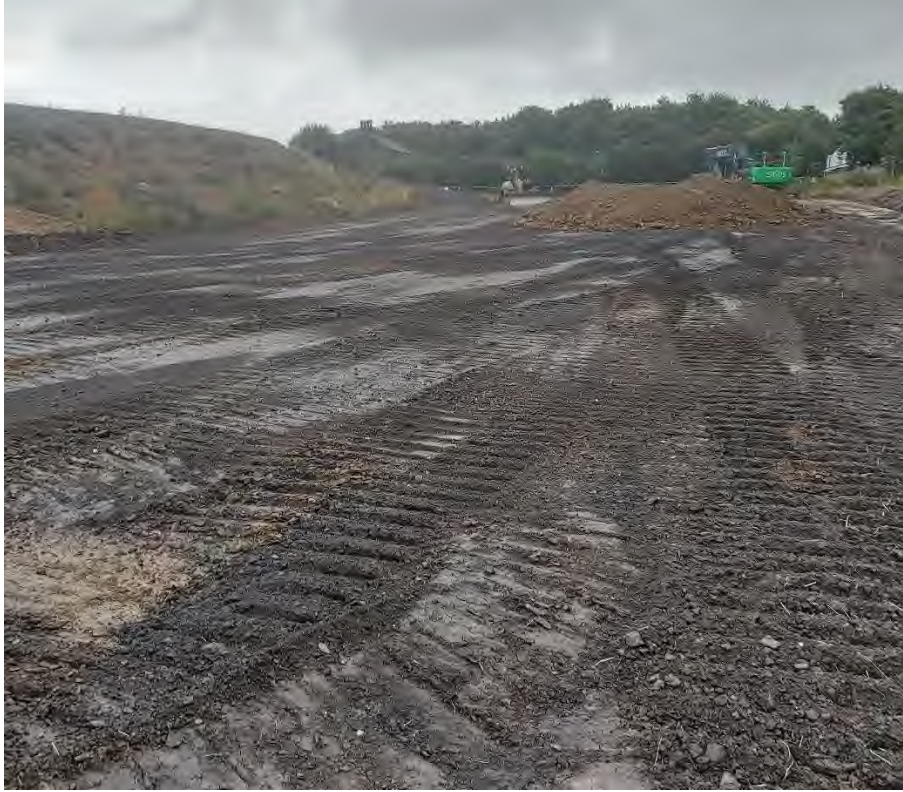
Photograph 01: Initial topsoil strip (17.07.23).
