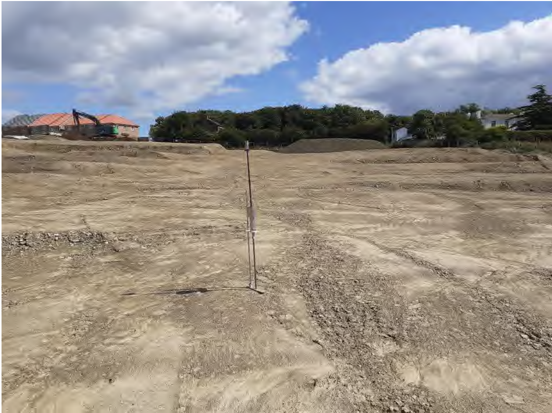
Photograph 14: Dynamic Cone Penetrometer testing of engineered ground within proposed highway (07.08.23).
