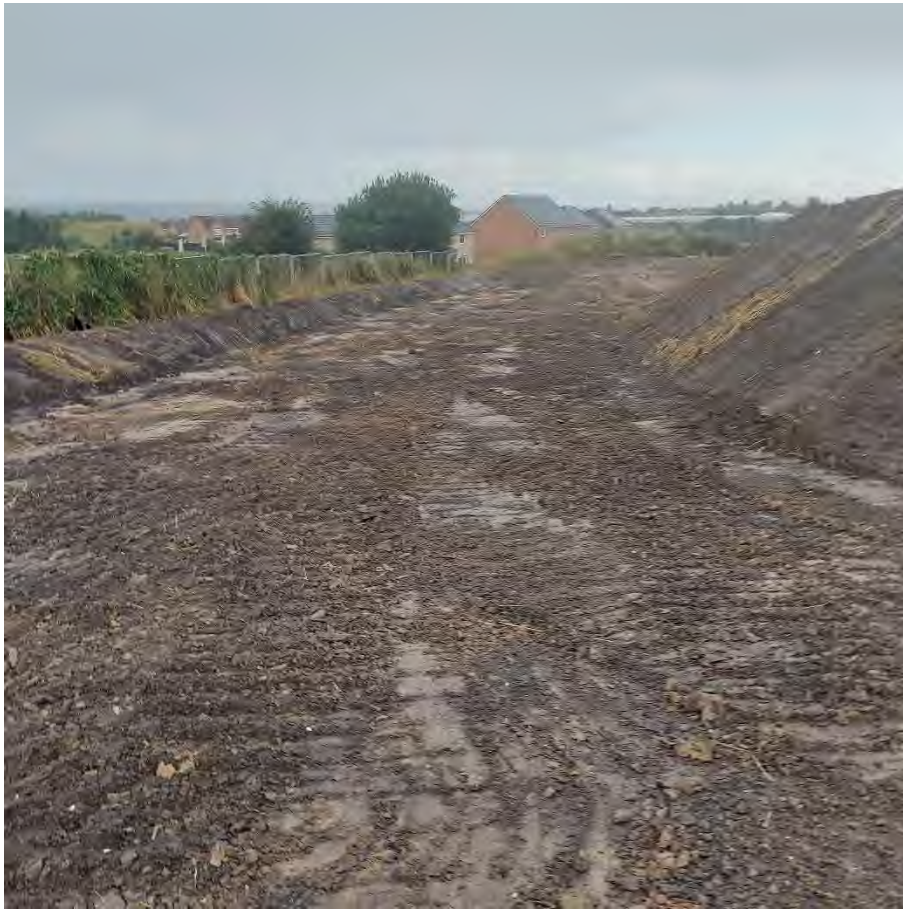
Photograph 02: Surface water runoff management bund located along the eastern boundary of the Phase 2 site (17.07.23).
