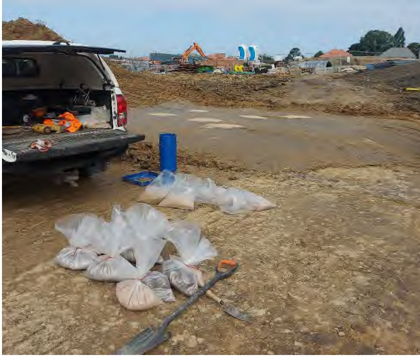
Photograph 05: Compaction Trial Pad on site-won fill (20.07.23).
