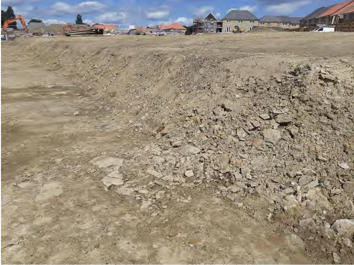
Photograph 16: Slope formed in cut separating plots 207-210 from plots 201-206 (08.08.23).
