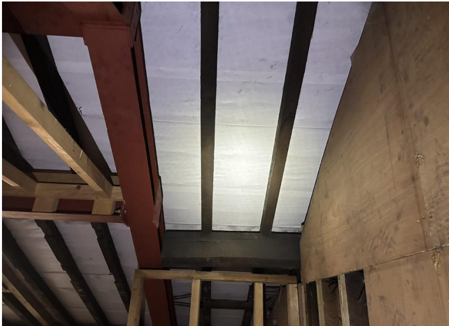
Photo 11. Modern, breathable roof felt, with little to no damage showing lack of suitability for roosting bats
