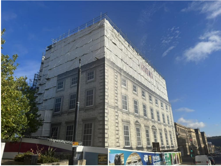
Photo 1. A typical view of the George Hotel (northeast aspect)
