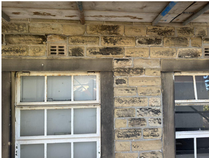
Photo 13. Close up shot of the George exterior, showing bricks, mortar, vent slots and window frames, in good condition
