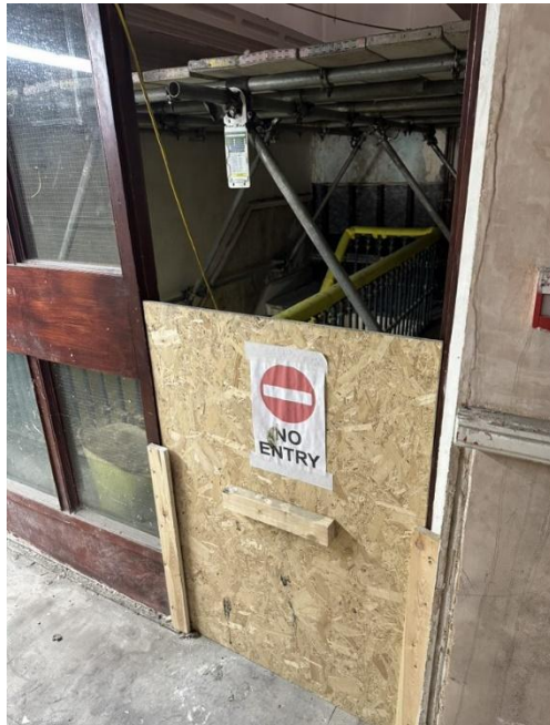
Photo 9. No entry sign to central staircase
