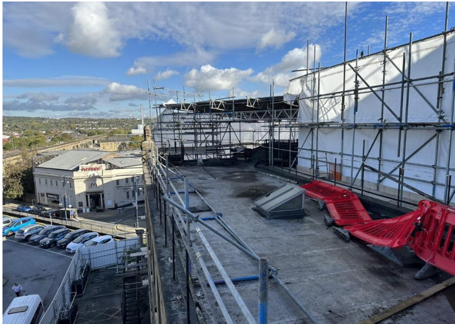
Photo 6. A section of the flat roof, facing north
