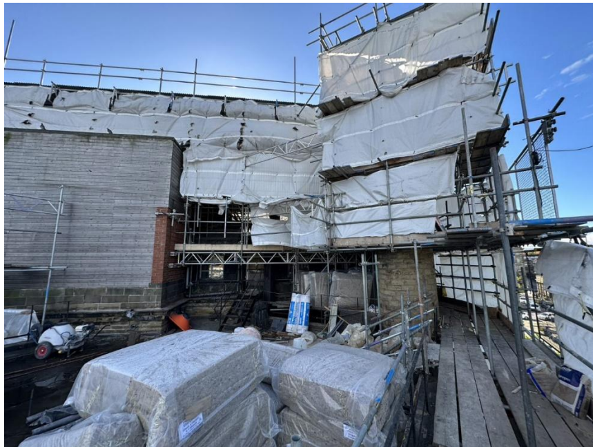
Photo 7. A section of the flat roof facing south
