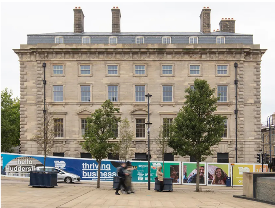
Figure 2 - Photo of Block A from St George's Square
