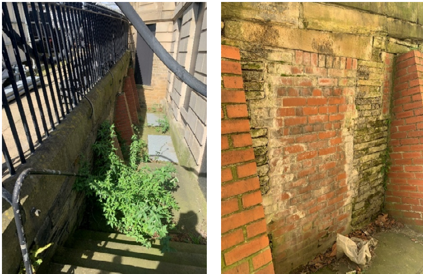
Figure 6 – Photos of Wall
