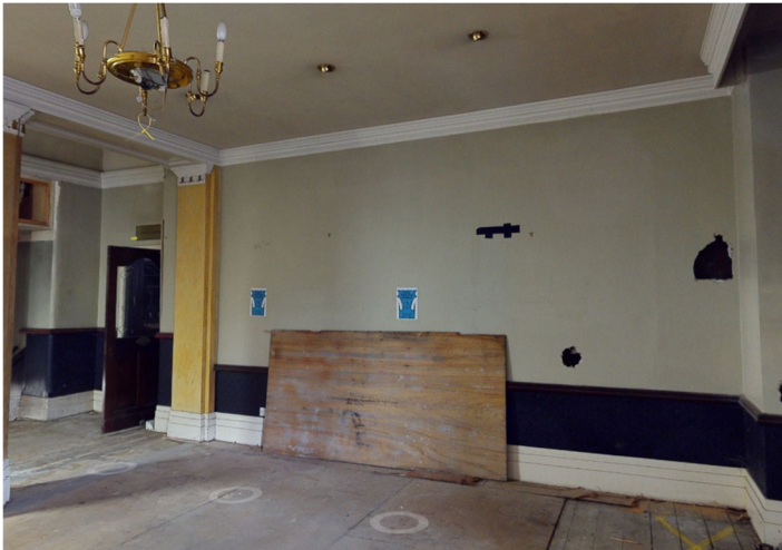
Figure 9 - Photo of Area to be Opened Up
