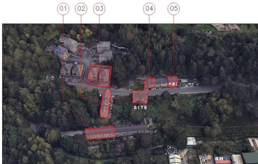
Aerial view of Proposed Site and surrounding properties.
