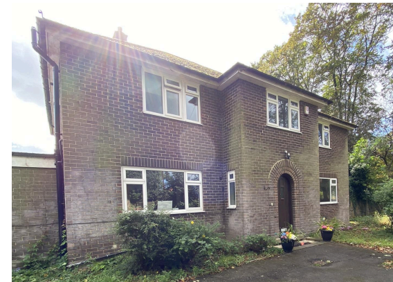
Existing vicarage to be demolished
