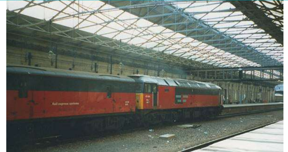
Figure 4.1.6b: Retained Roof A lighting scheme in 1990s
