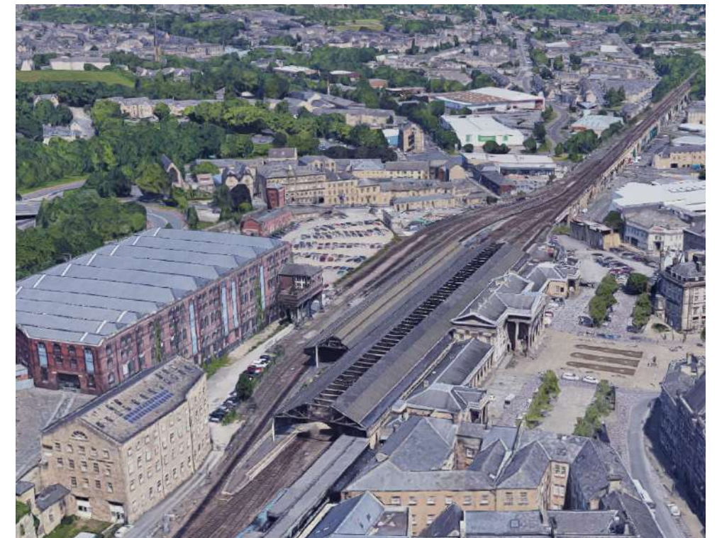
Figure 2.1d: Looking north over Huddersfield viaduct
