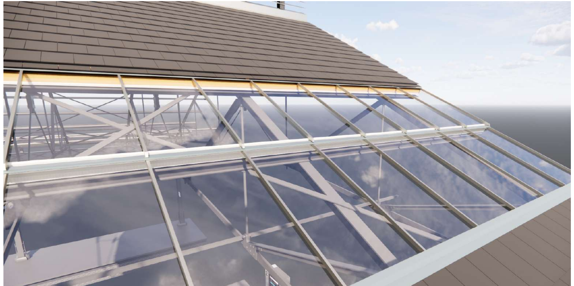
Figure 4.2.2a: Visual showing polycarbonate rooflights
