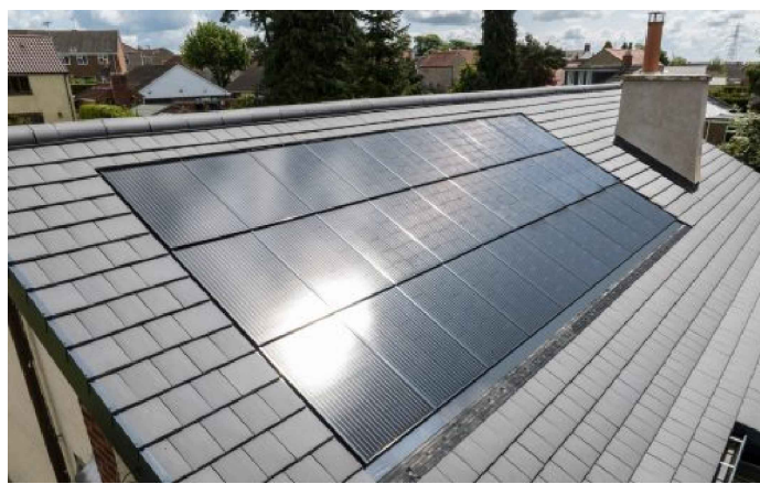
Recessed Solar Panels Scale NTS
