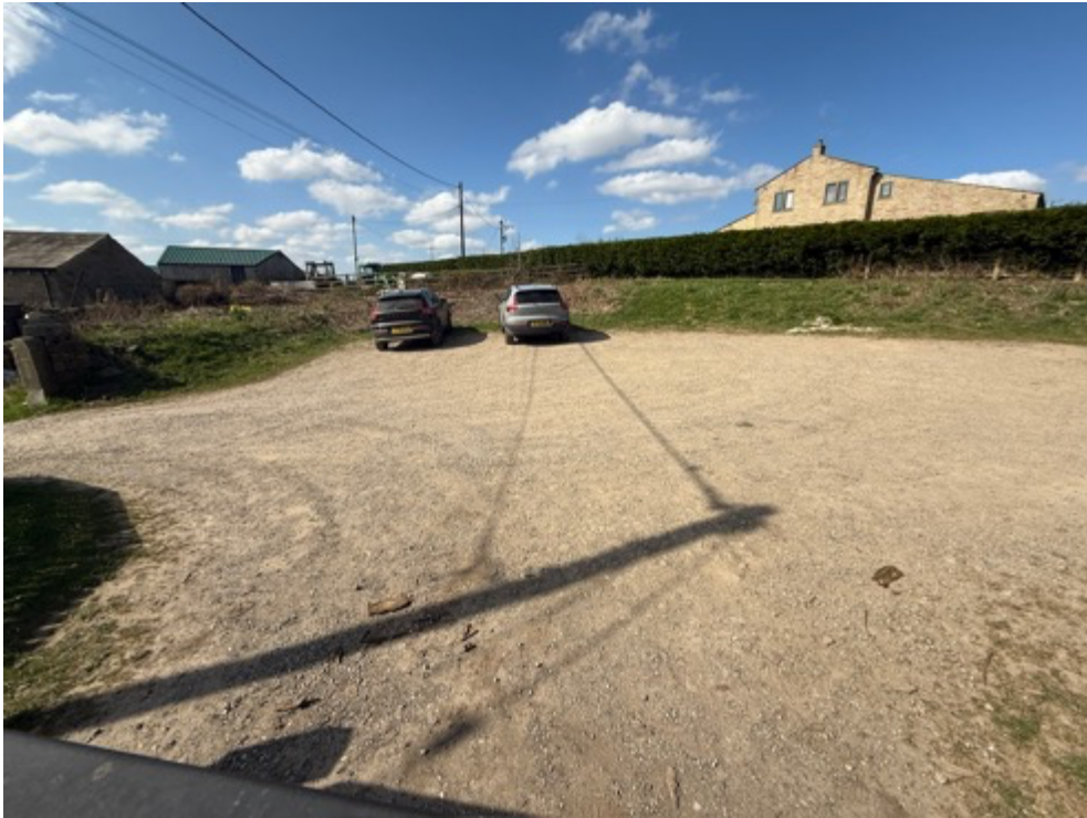
Unsealed surface that forms the access track through the site.
