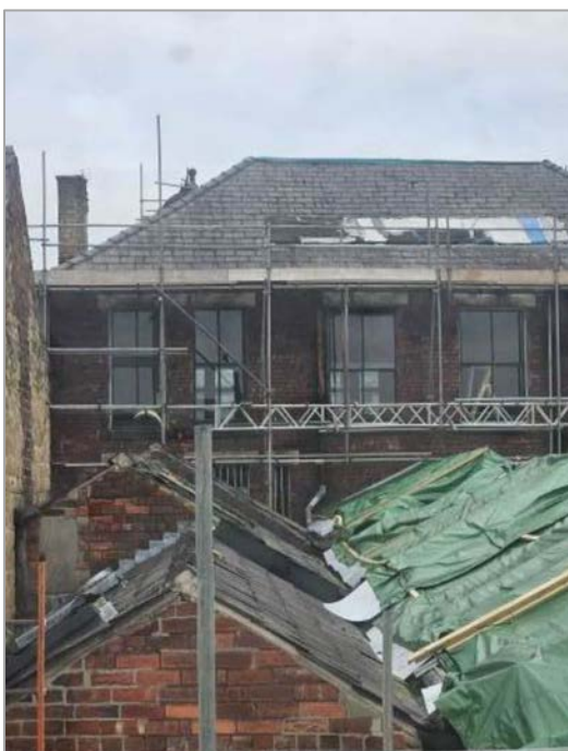
Figure 4.2: South roof of the northern entrance building (Jan. 2025)
