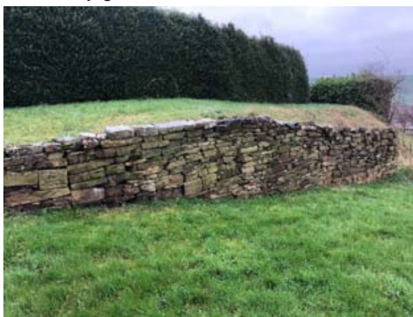
Photograph 7—Dry Stone Revetment Wall
