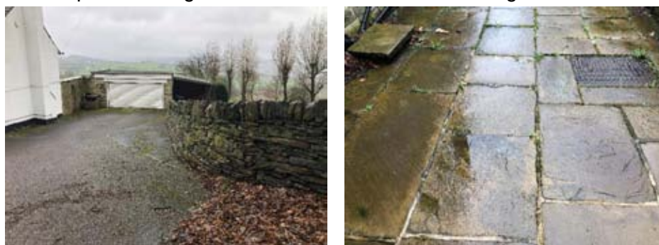
Photograph 3 and 4—Hard Surfaced driveway and stone flags with mortared joints
