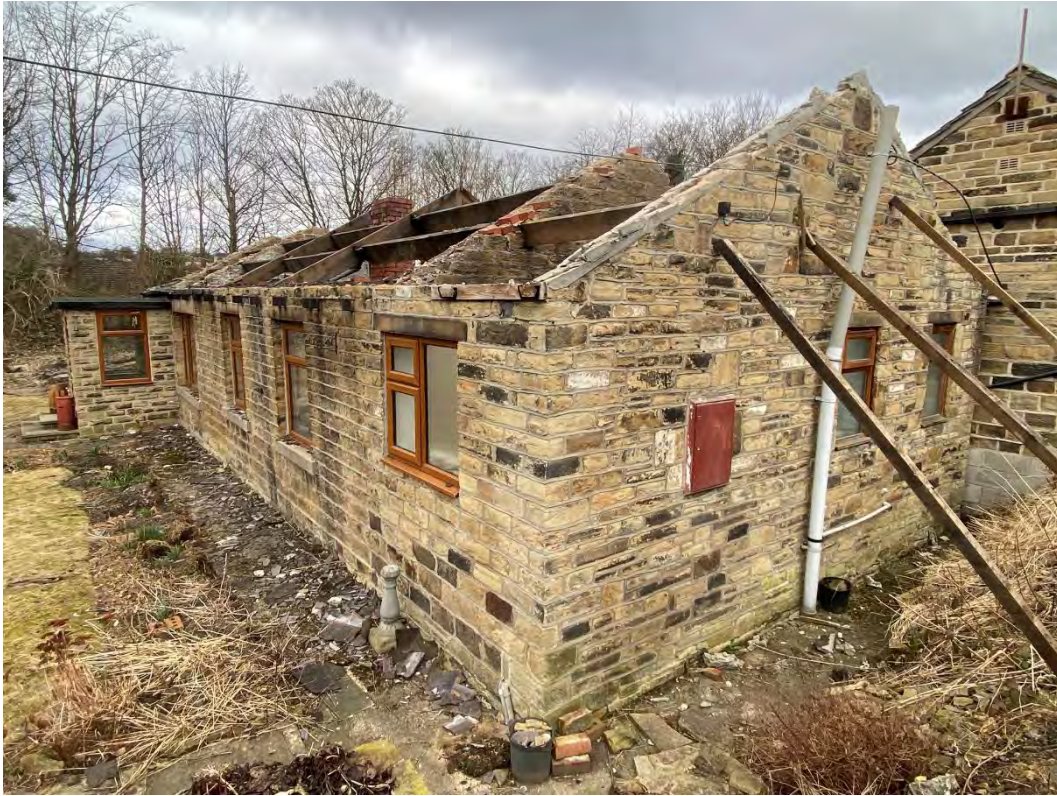
Photo 5. House viewed from south-east
