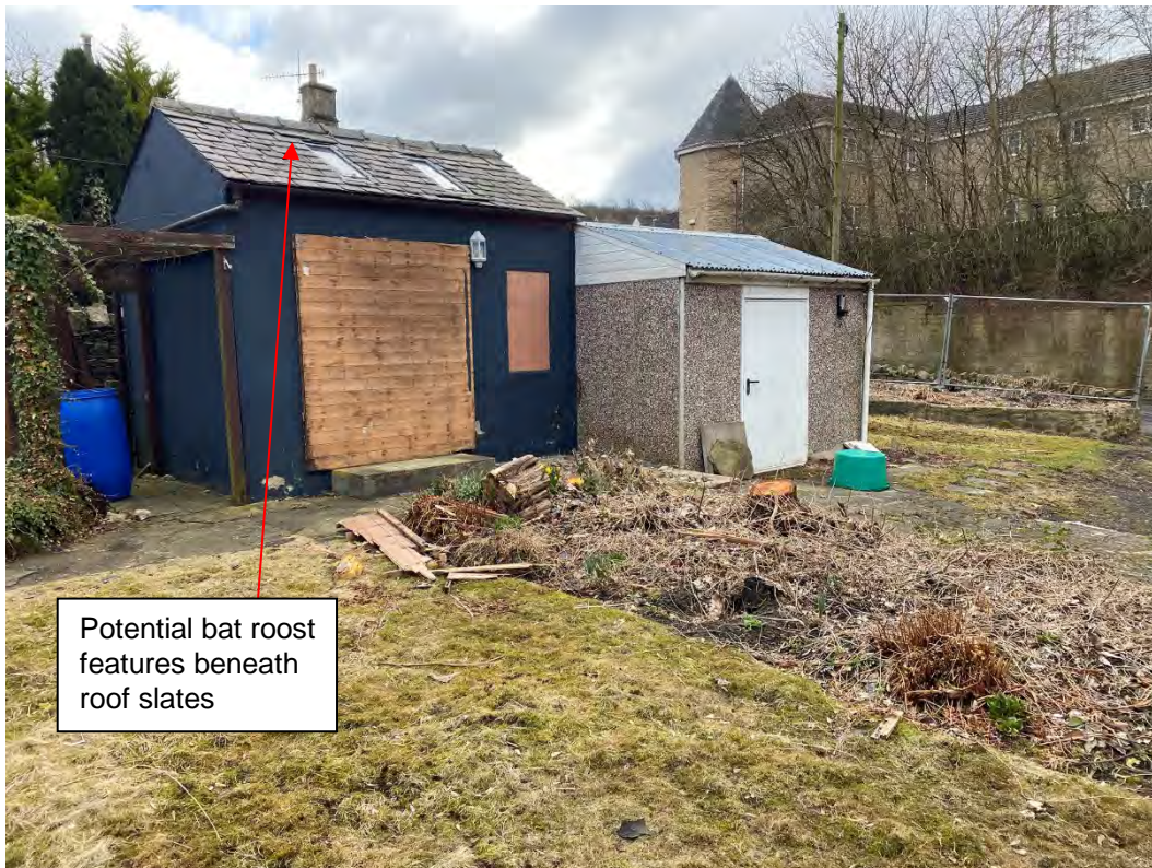
Photo 8. Outbuildings viewed from north-west
