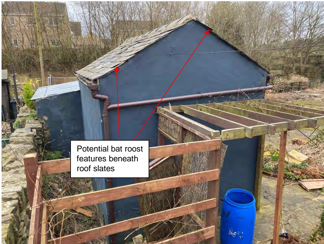
Photo 10. Outbuildings viewed from north
