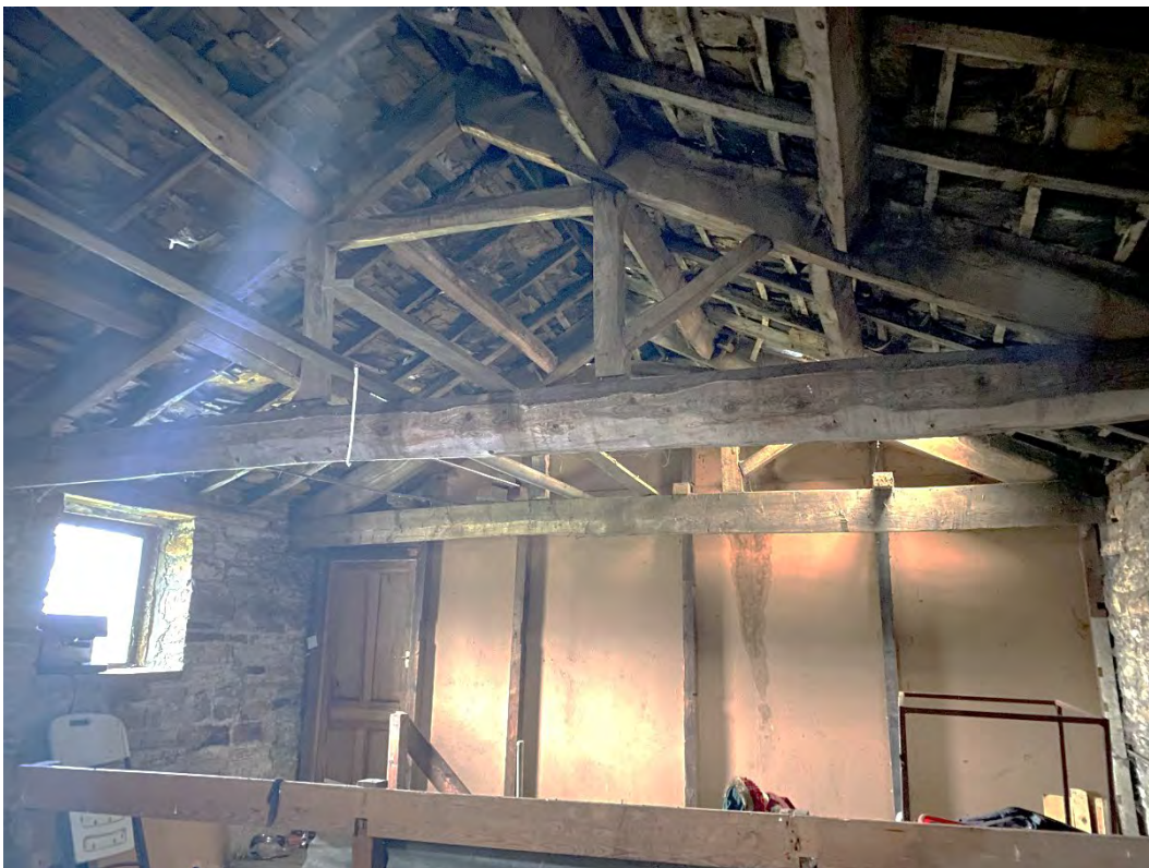
Photo 10. Interior of barn – first floor - looking north
