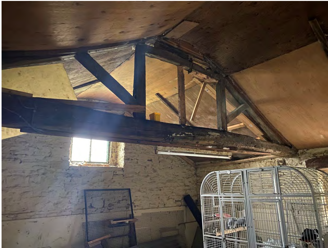
Photo 11. Interior of barn – first floor – looking towards north gable
