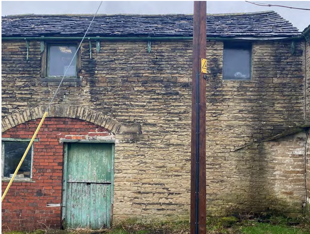
Photo 7. Barn – west elevation
