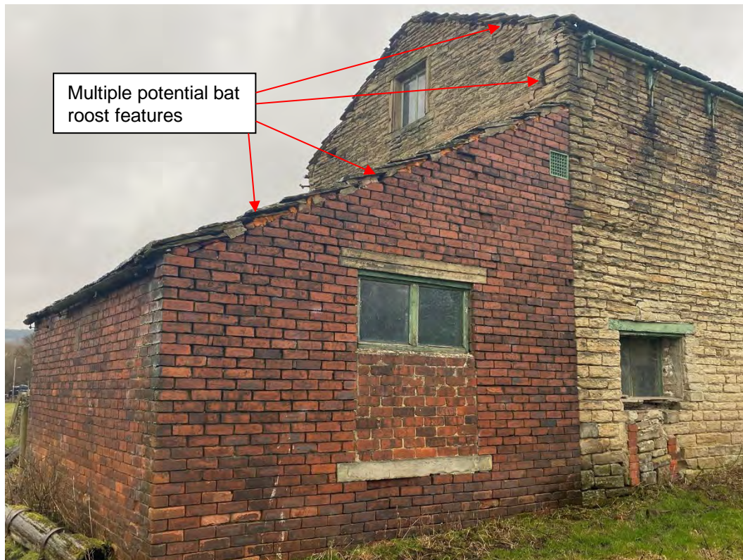
Photo 4. Barn viewed from north-west
