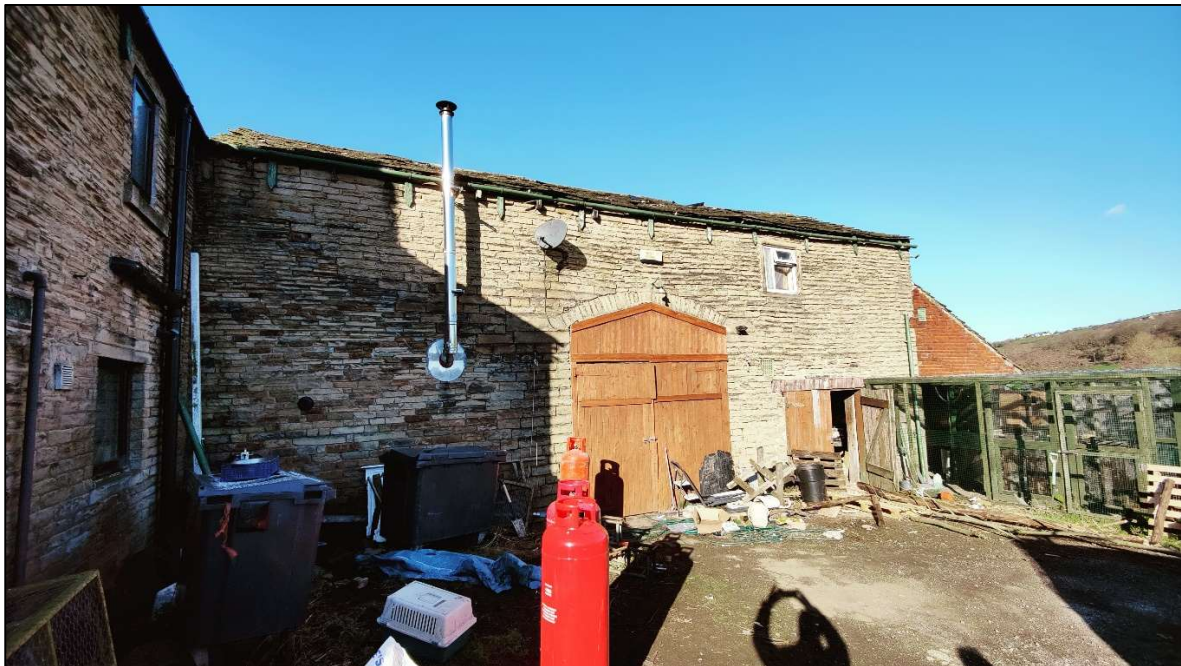
East elevation of the attached barn subject to this application
