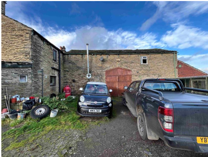
Photograph 1 – Barn East Elevation
