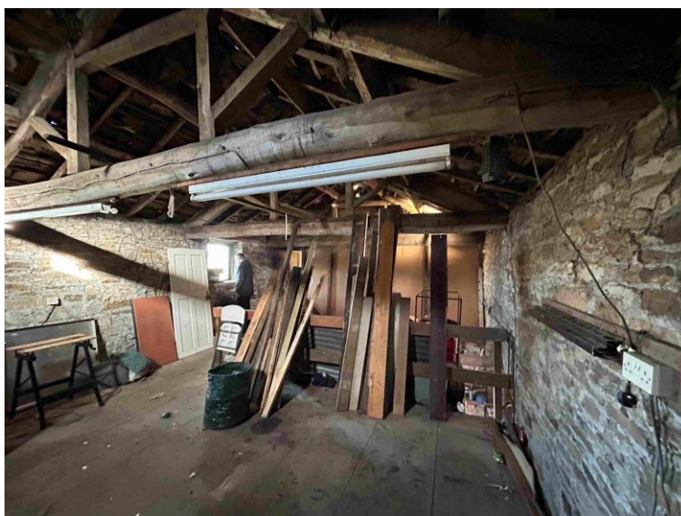
Photograph 5 – Main Roof Structure
