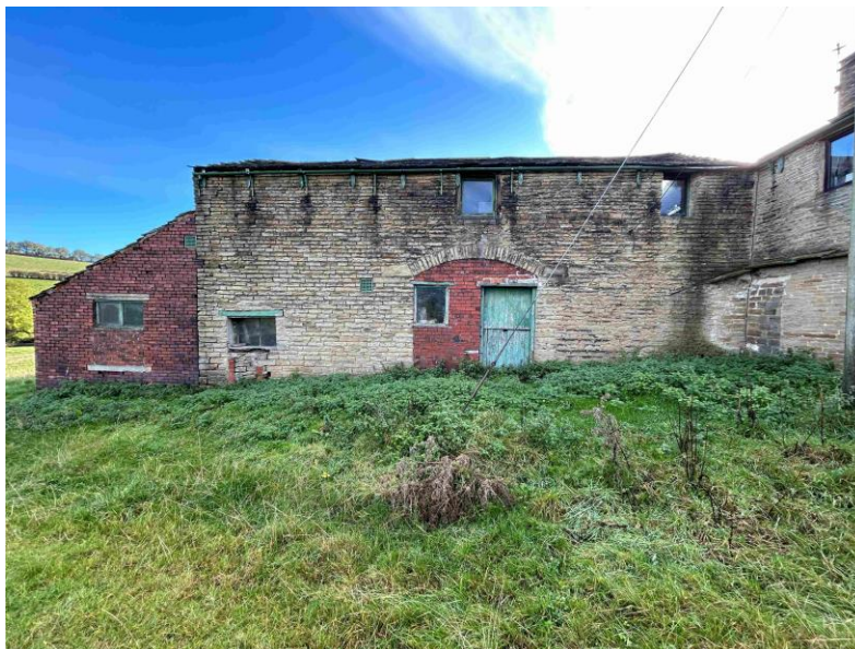
Photograph 2 – Barn West Elevation
