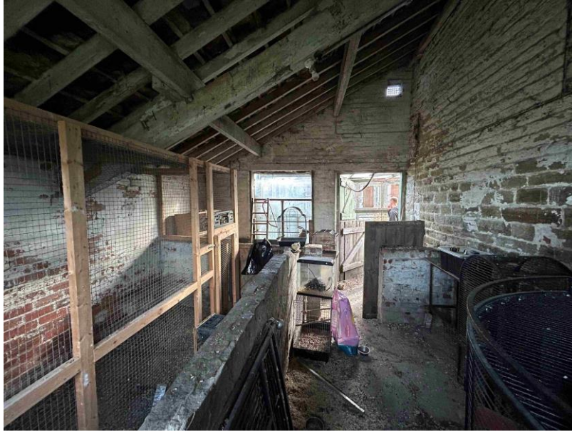
Photograph 6 – ‘Lean To’ Roof Structure
