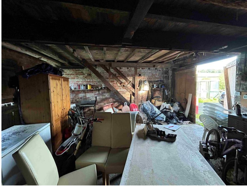
Photograph 7 – First Floor Structure in Main Barn.
