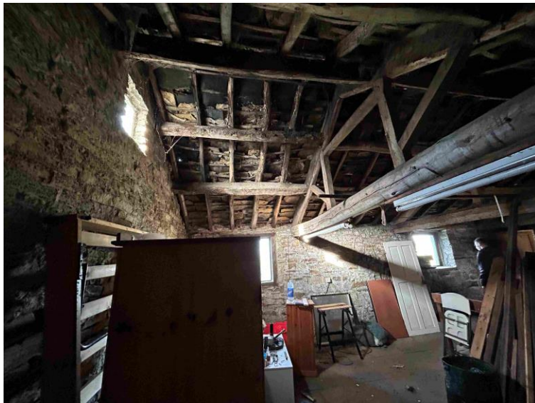
Photograph 4 – Main Roof Structure
