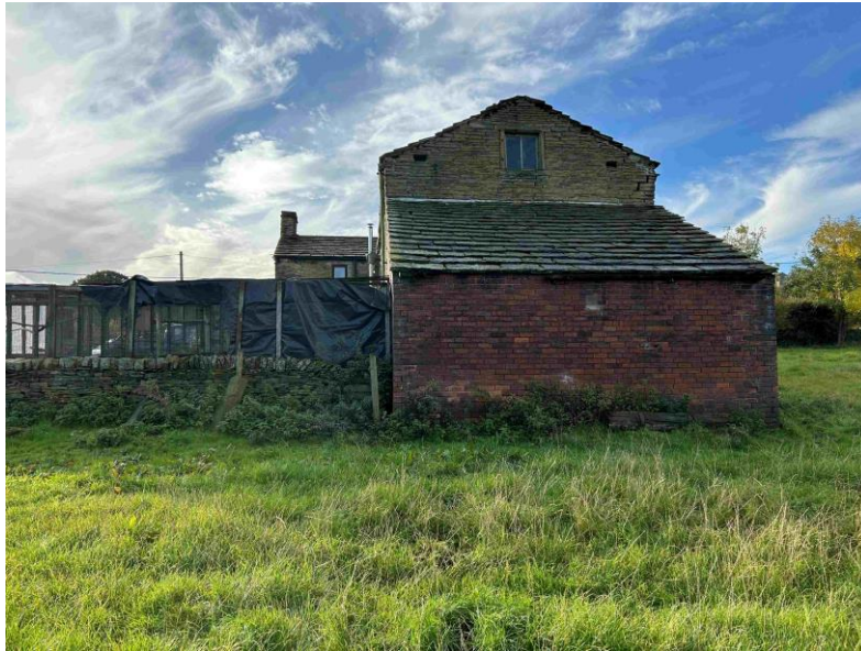
Photograph 3 – North 'lean to' section
