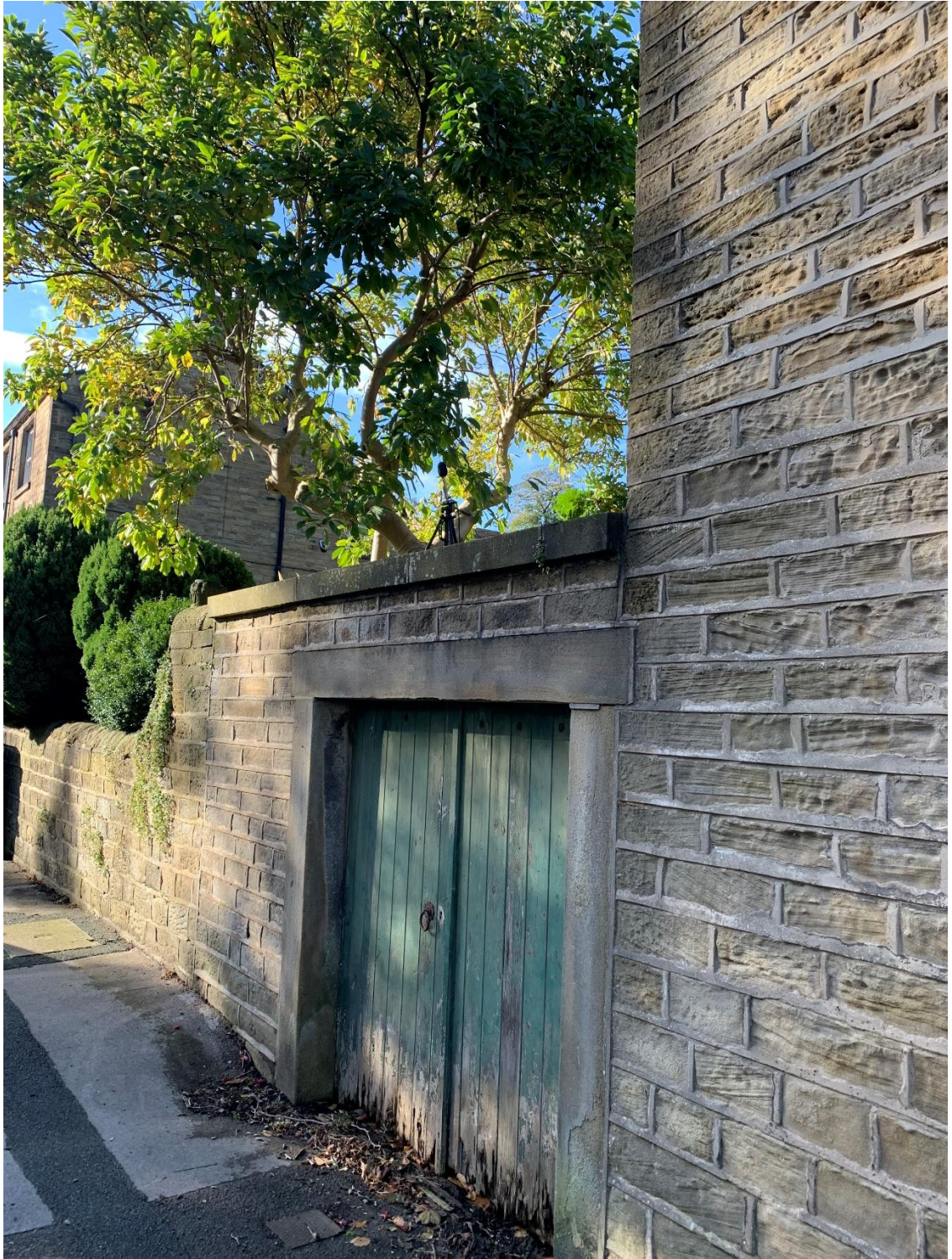
Existing stable access door off Woodhead Road
