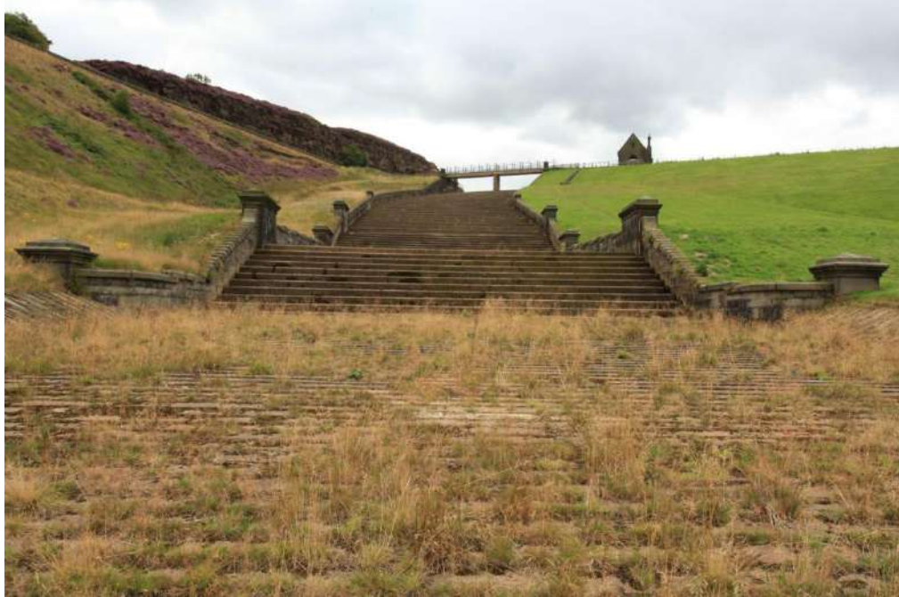
Figure 3: Spillway at Butterley Reservoir
