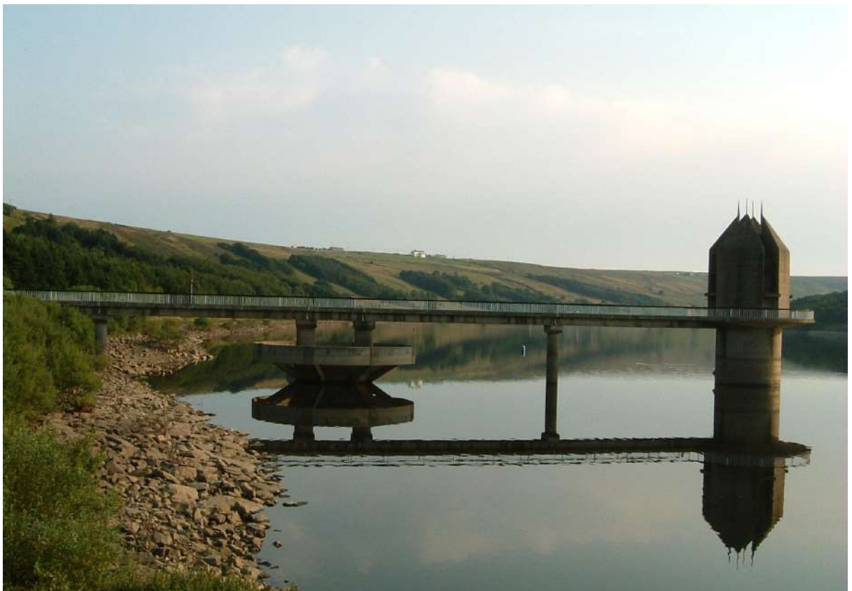
Figure 8: Pumphouse at Scammonden Reservoir
