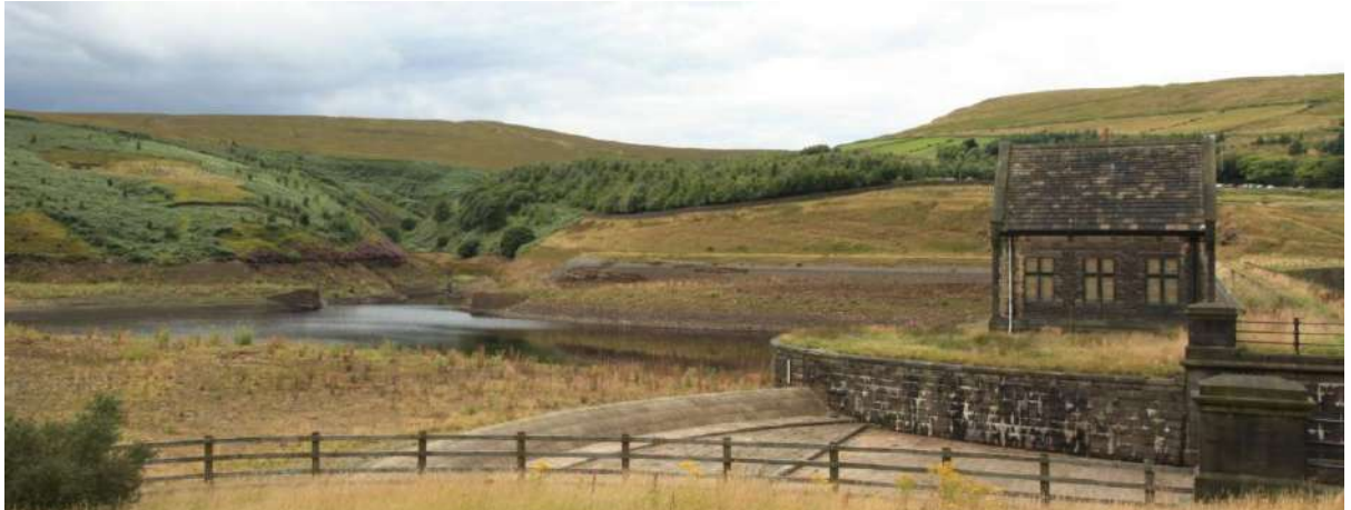
Figure 7: Pumphouse at Butterley Reservoir
