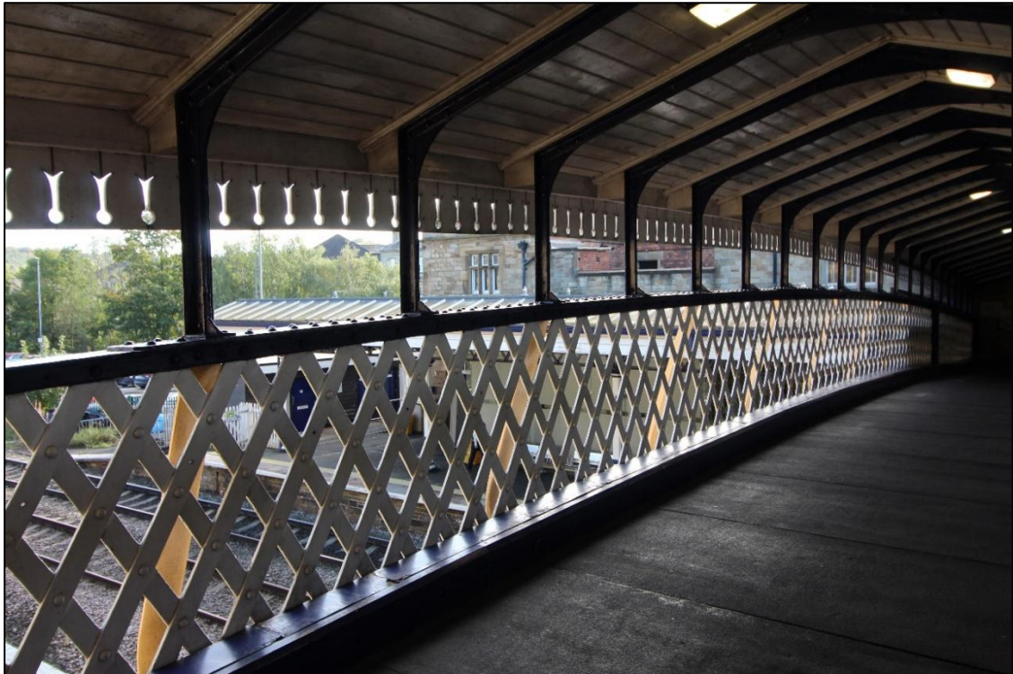
Plate 24: Northern elevation of footbridge looking north-east, (IMG_2169)
