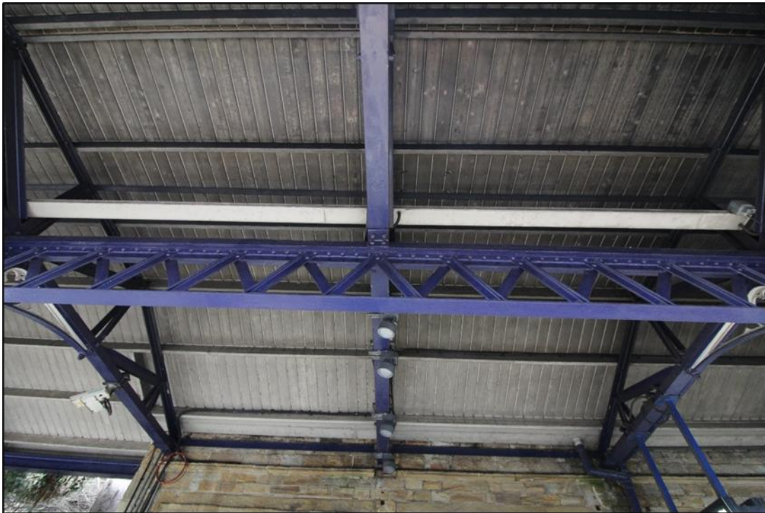
Plate 6: Underside of Platform 1 canopy roof, timber panelling, looking west (IMG_2207)
