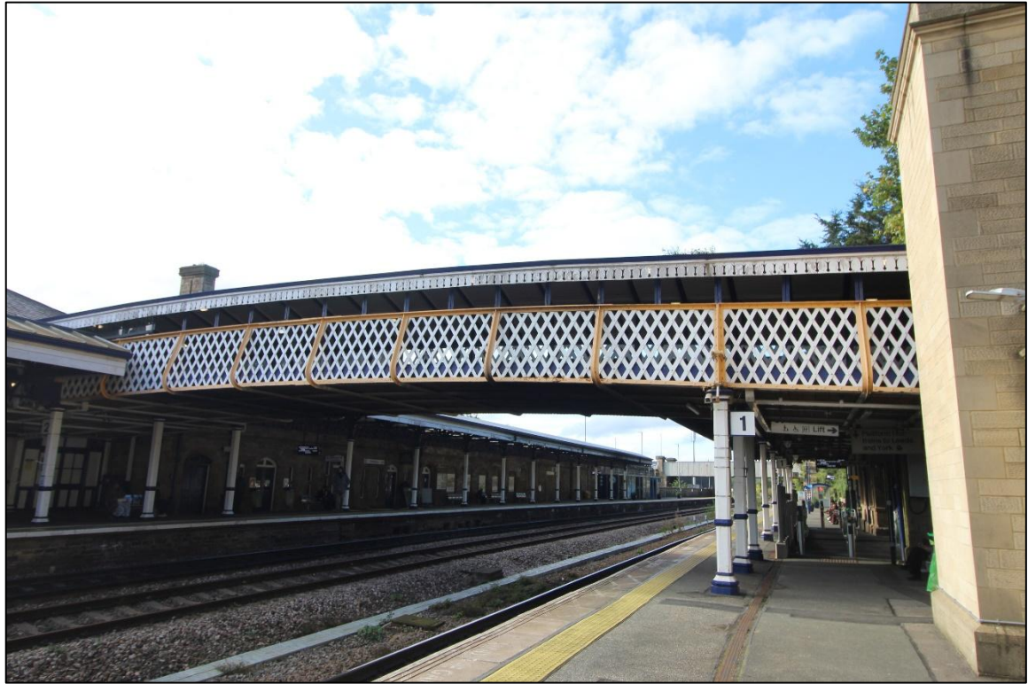
Plate 18: Northern elevation of footbridge (from Platform 1), looking south-east, (IMG_2190)
