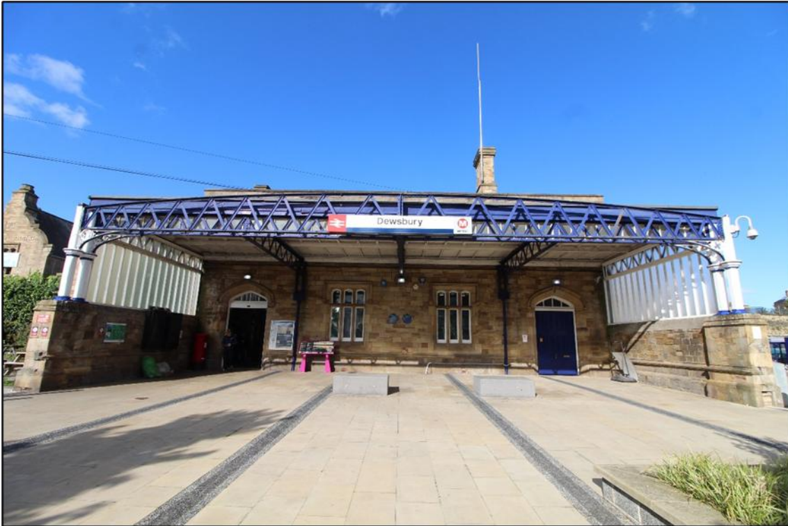
Plate 4: Exterior of Dewsbury Station (MDL1/18) entranceway, eastern elevation (IMG_2296)
