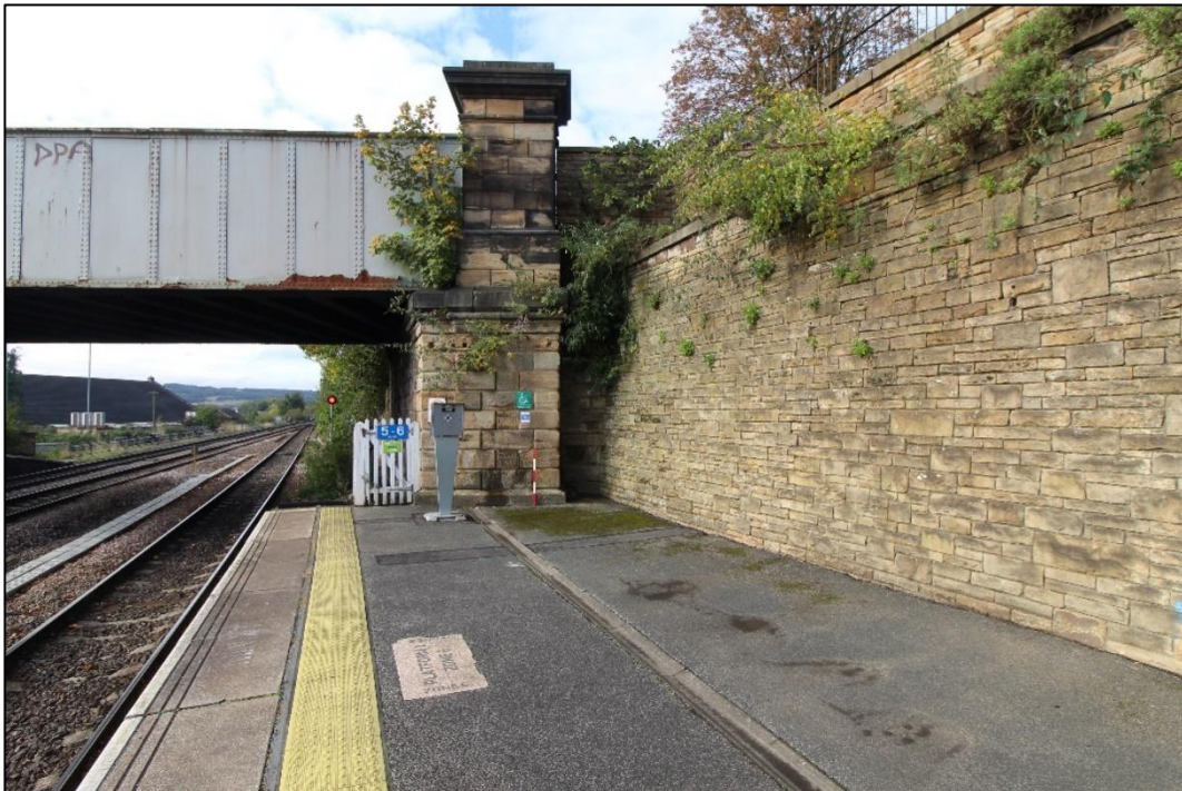
Plate 11: Southern end of platform 1, showing retaining wall, 1m scale, (IMG_2241)
