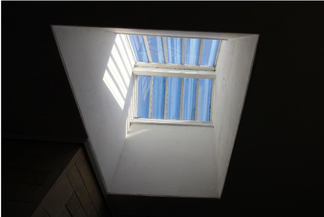
Plate 22: Skylight on eastern end of footbridge, (IMG_2279)
