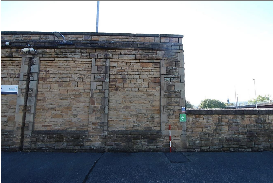
Plate 15: Southern end of Platform 2 retaining wall, looking east, 1m scale, (IMG_2105)
