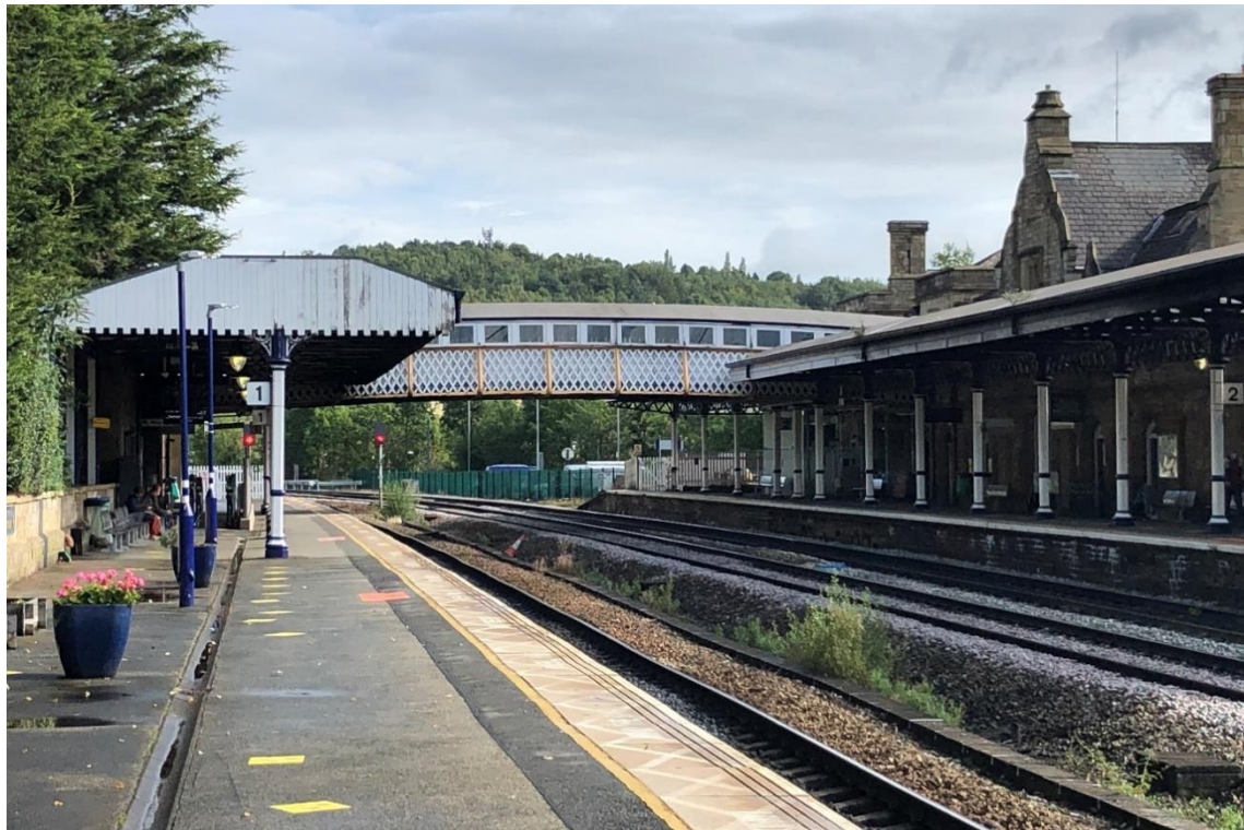
Insert 4-3 Dewsbury Station platform, showing platform canopies and footbridge.
