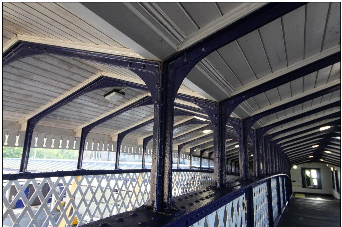
Plate 25: Central partition and pointed roof of footbridge, looking east (IMG_2151)
