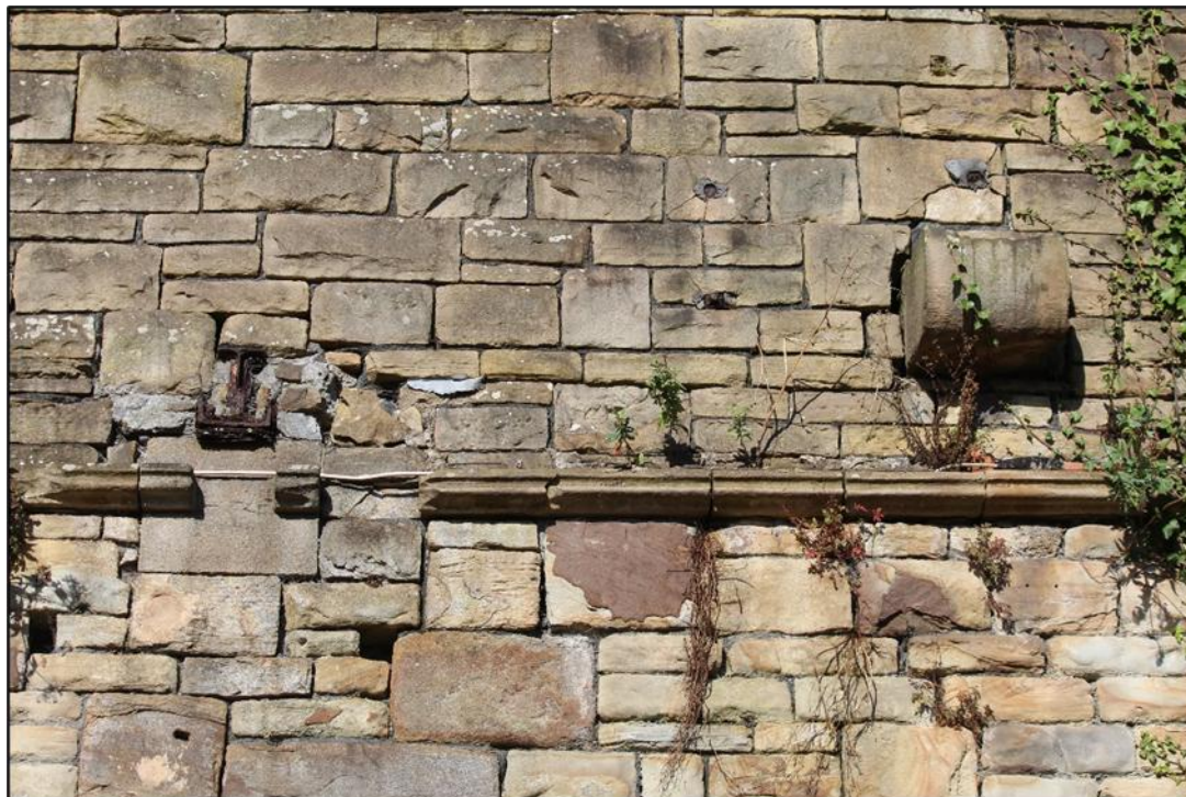
Plate 12: Northern end of platform 1 retaining wall features, looking east, (IMG_2263)
