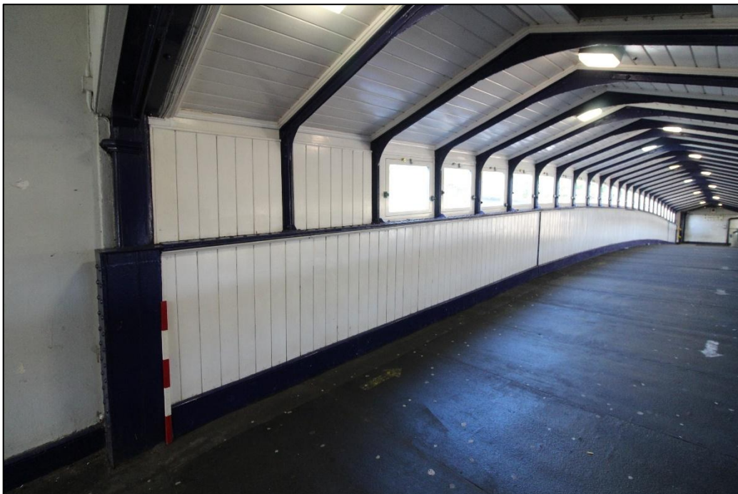
Plate 23: Windows on Southern elevation of footbridge looking south-west, 1m scale (IMG_2139)
