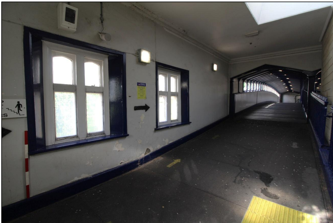
Plate 21: Windows on eastern end of footbridge, looking south-west, 1m scale (IMG_2268)
