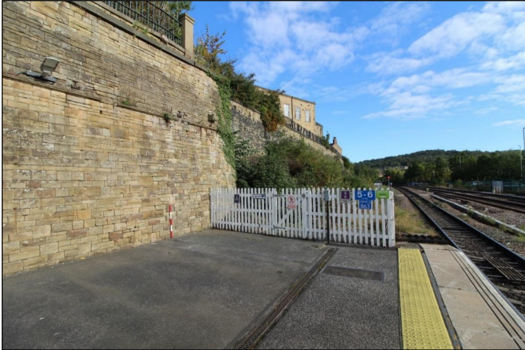
Plate 10: Northern end of platform 1, showing retaining wall, 1m scale, (IMG_2188)
