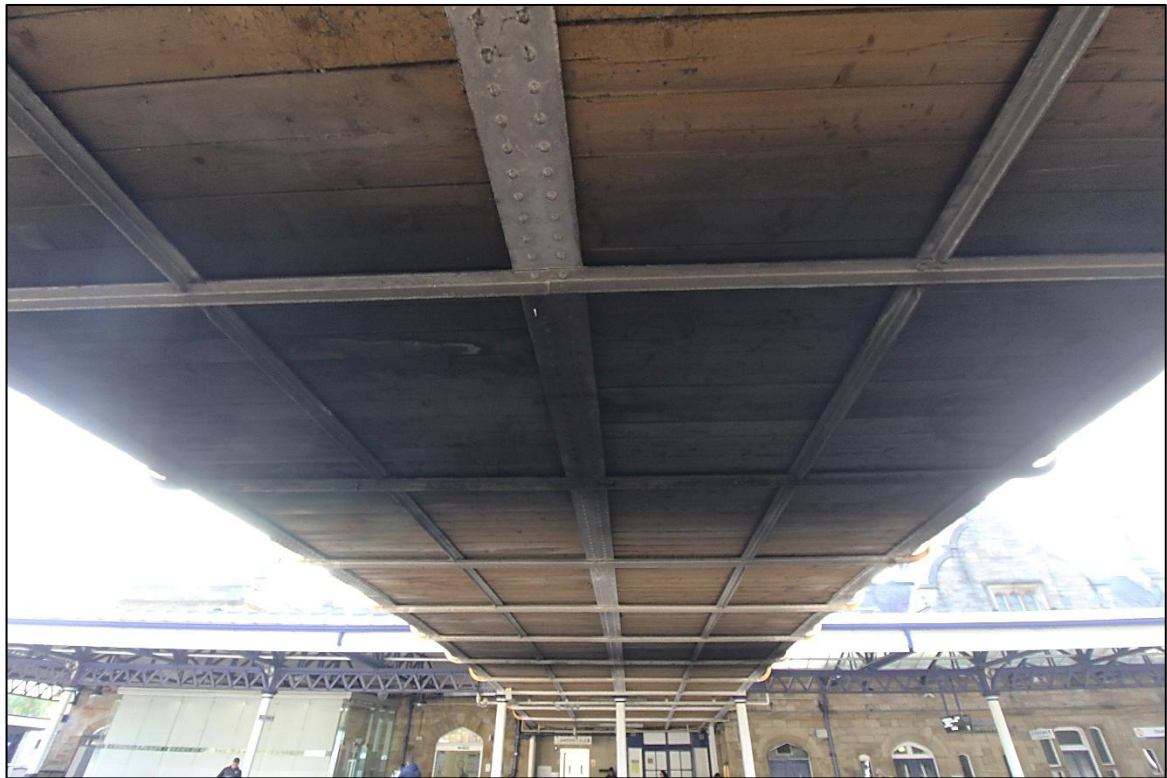
Plate 19: Underside of footbridge, looking east, (IMG_2219)
