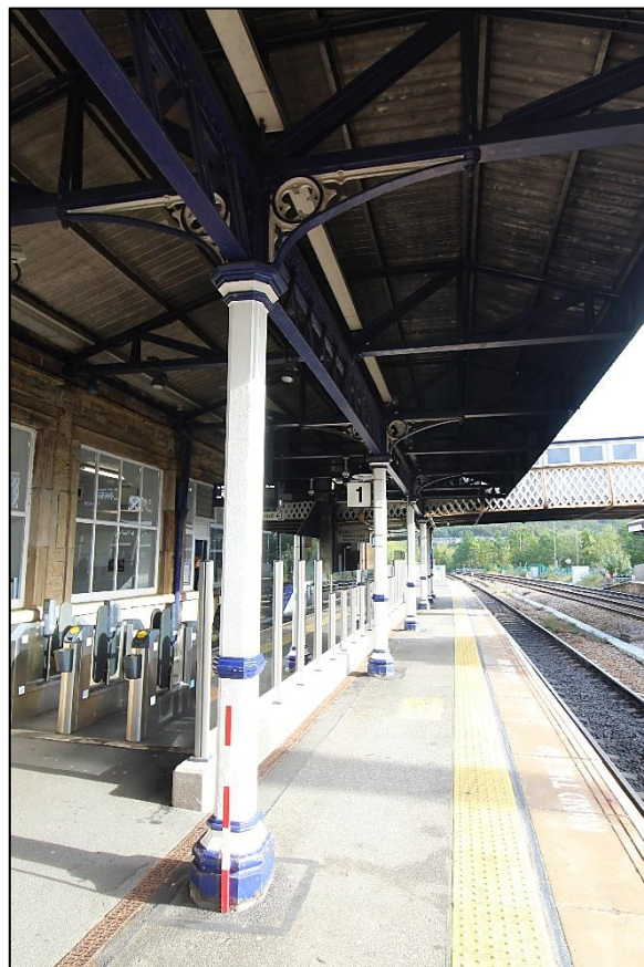
Plate 7: Platform 1, cast-iron columns and brackets, 1m scale, looking north, (IMG_2202)
