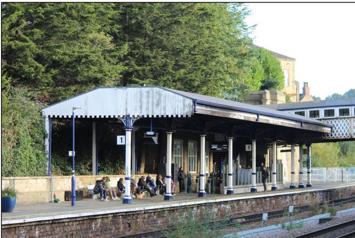
Plate 5: Dewsbury Station (MDL1/18) Platform 1 canopy. View facing north-west (IMG_2080)
