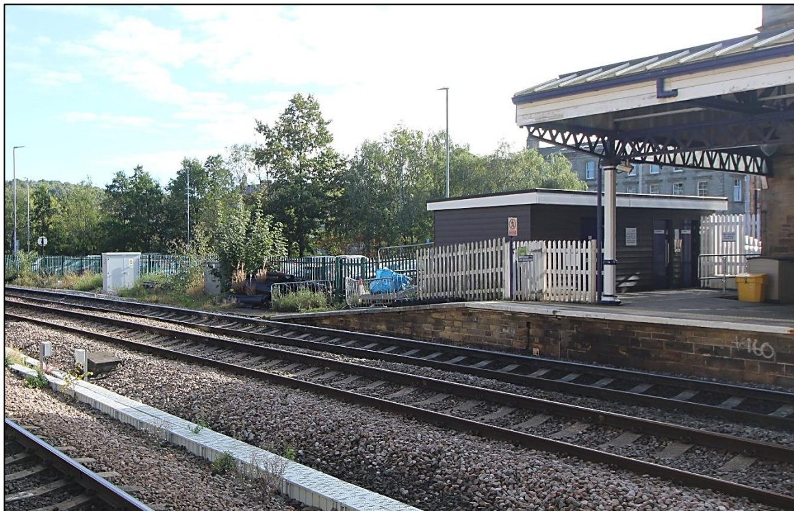
Plate 16: Northern end of Platform 2, looking north-east, (IMG_2186)
