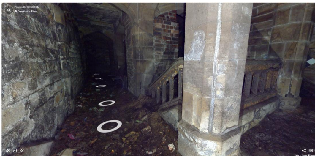
Plate 29: View north from north-western extent of subway area (screenshot from 3D model provided by client)
