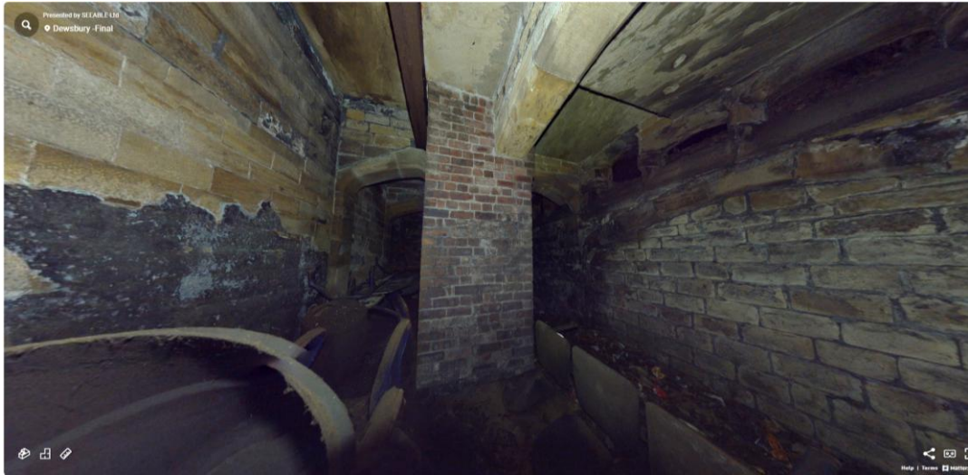
Plate 33: Southern part of subway area showing brick-built column opposite blocked central archway in western wall (screenshot from 3D model provided by client)
