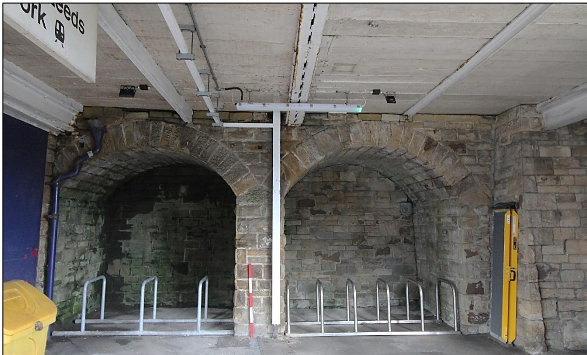
Plate 8: Platform 1, cast-iron downpipe (to left) and archways, 1m scale, (IMG_2224)
