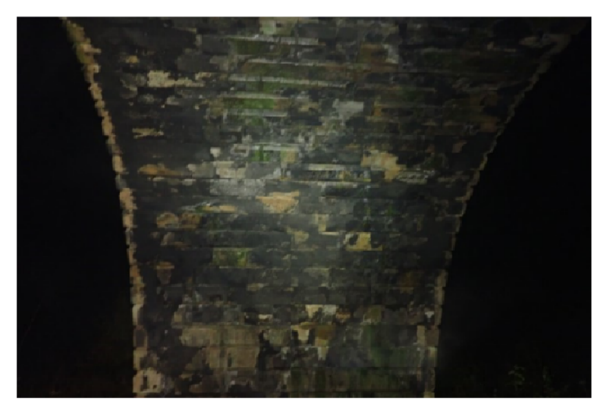
Photo 2: General Soffit View
