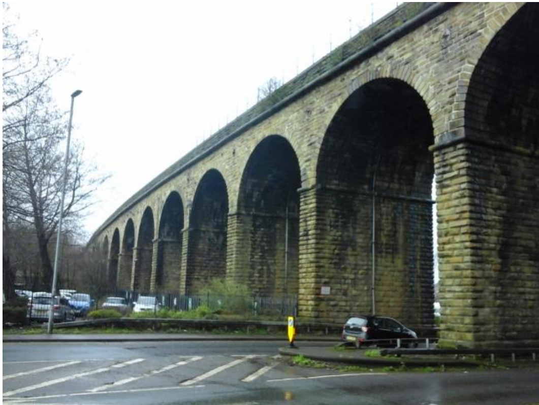
Insert 4-3 Upper Mill (Batley) Viaduct (MDL1/27), eastern elevation looking south.
