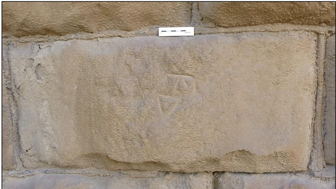
Plate 16: Example of mason's mark on southern pier of Span 6 with 50mm scale. View facing south (0500.JPG)
