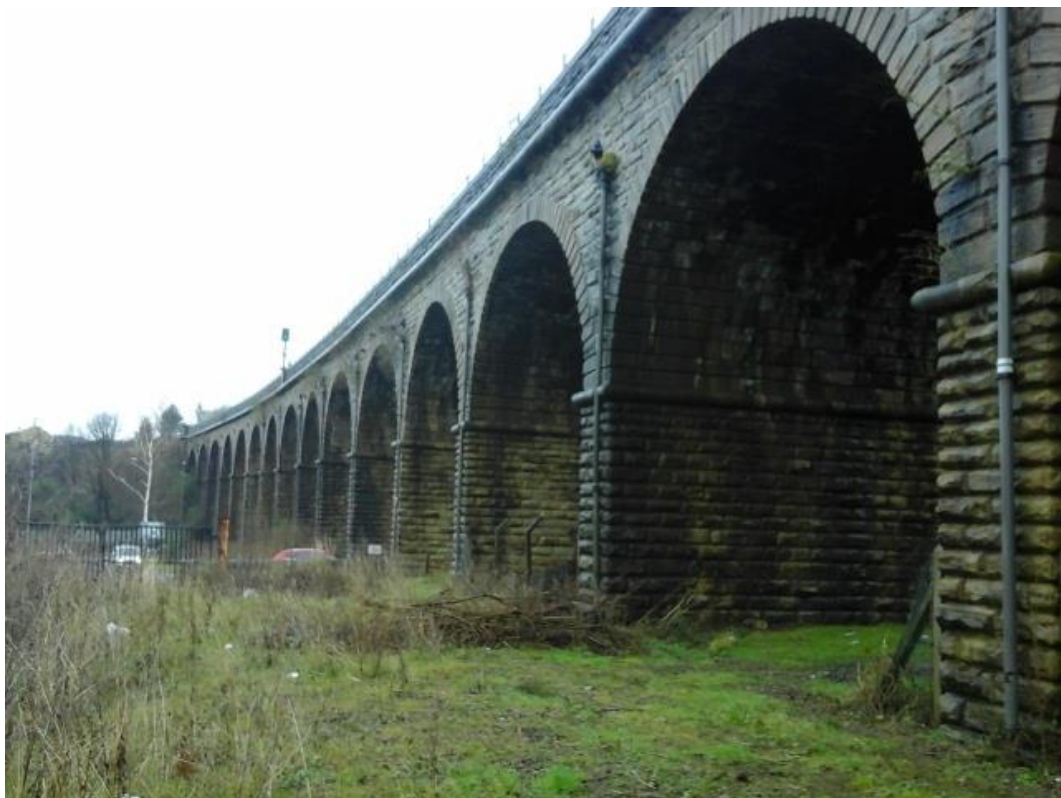
Insert 4-4 Upper Mill (Batley) Viaduct (MDL1/27) western elevation looking north.
