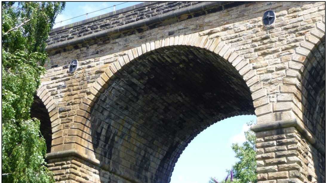
Plate 7: Spring of Span 12. View facing north-east (0472.JPG)
