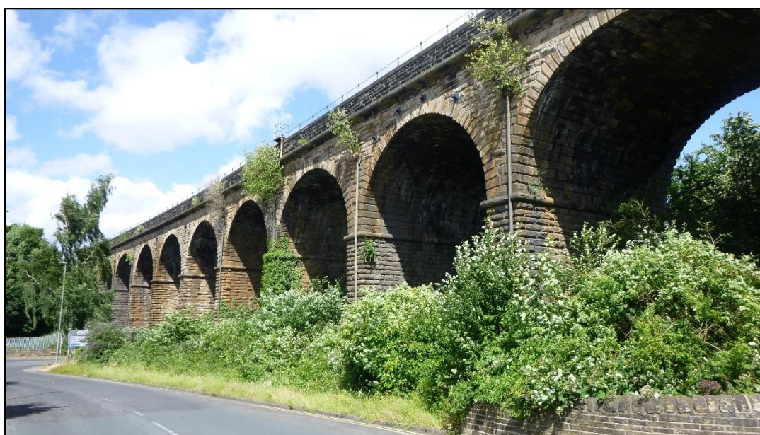
Plate 3: Northern end of western elevation. View facing north-east (0483.JPG)
