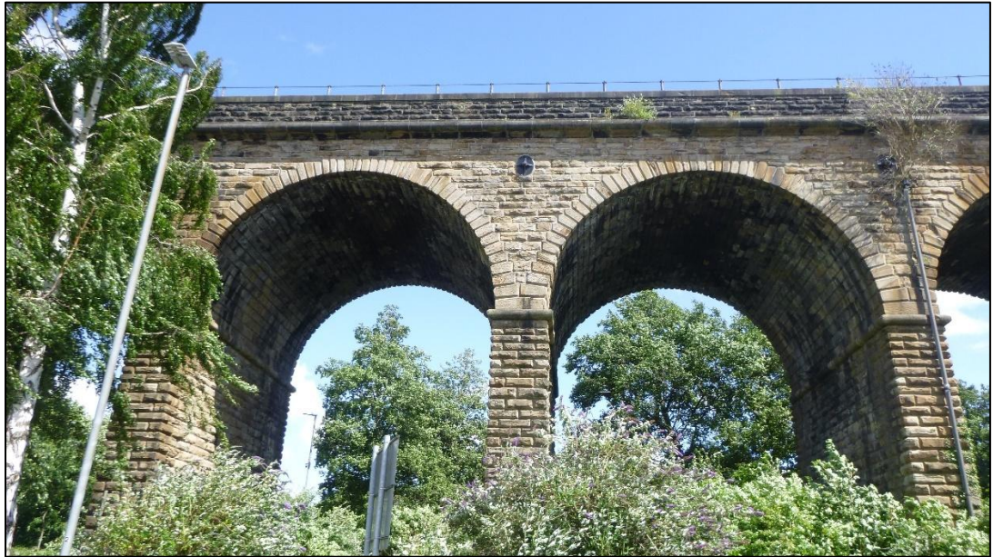
Plate 6: Spans 11 and 12. View facing east (0471.JPG)
