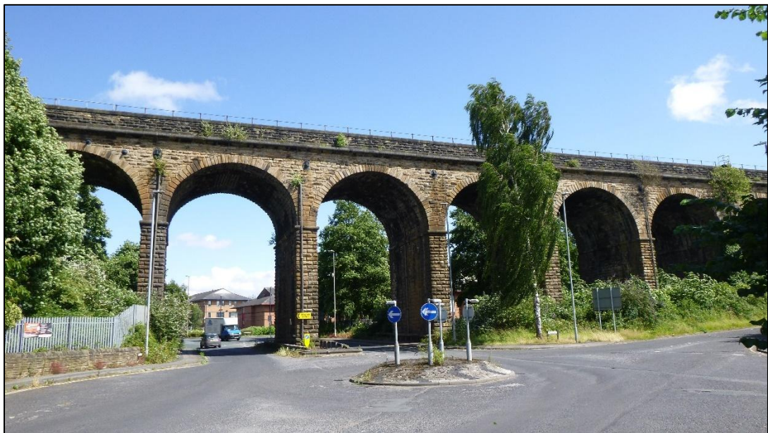
Plate 5: Northern end of western elevation. View facing east (0505.JPG)
