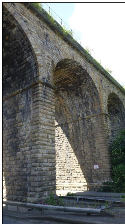
Plate 11: Span 14 on eastern elevation. View facing north-west (0499.JPG)
