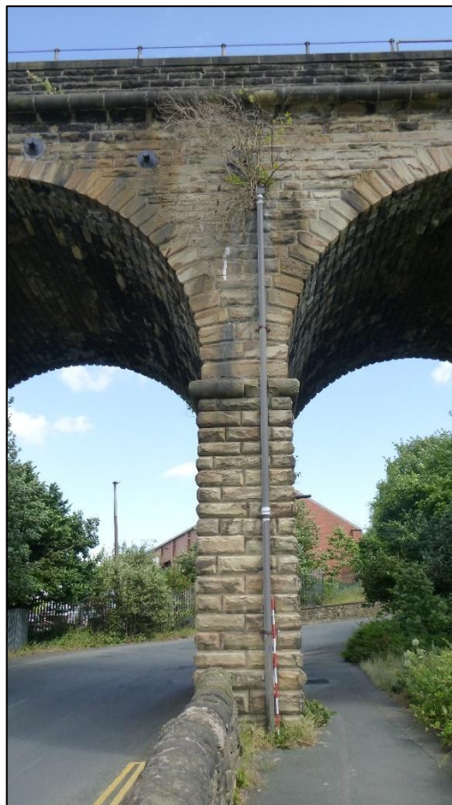
Plate 9: Pier between Spans 5 and 6. With 2m scale. View facing east (0484.JPG)
