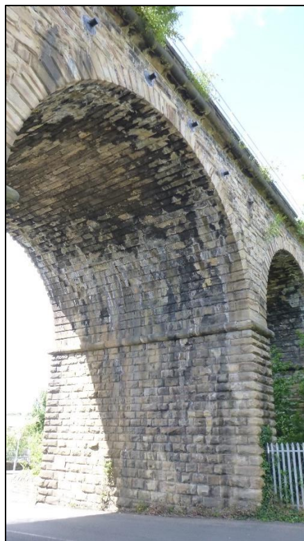
Plate 13: Internal space of Span 6. View facing north-west (0489.JPG)
