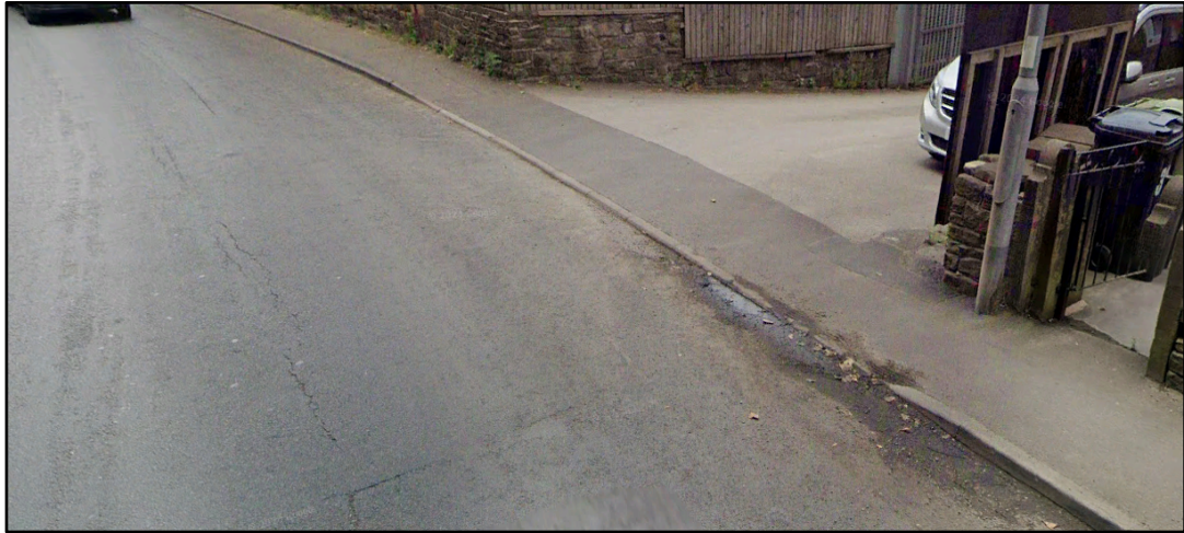
Figure 2.1 Photograph of Existing Site Access
