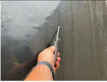
Pick testing along adherence between adjacent sheets of Juta TitanTank.
