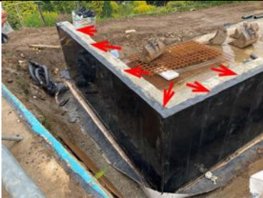
Evidence of Juta GP Primer applied to the retaining wall.
