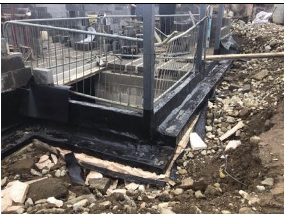
Perimeter retaining wall tanking detail
