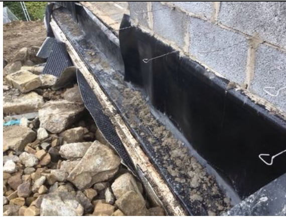
Perimeter retaining wall tanking detail
