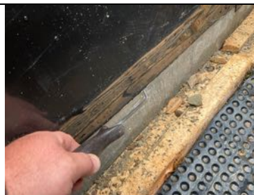
Pick & probe testing along termination to existing Juta TitanBond gas barrier.
