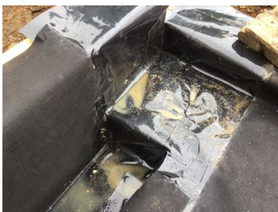
Corner detailing sealed using Juta Titan tank and heat applied
