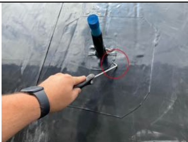
Pick testing to the sealed water pipe.
