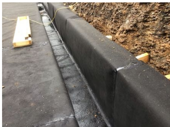
Membrane extended over the perimeter edge shuttering
