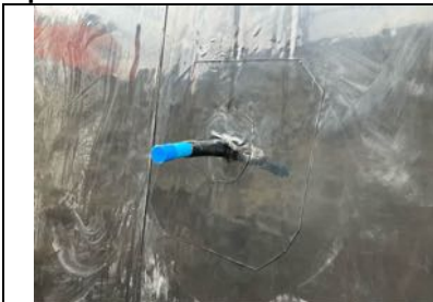
25mm Water Pipe sealed using Juta TitanTank.
