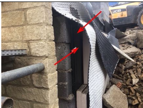
Existing previously installed tanking
