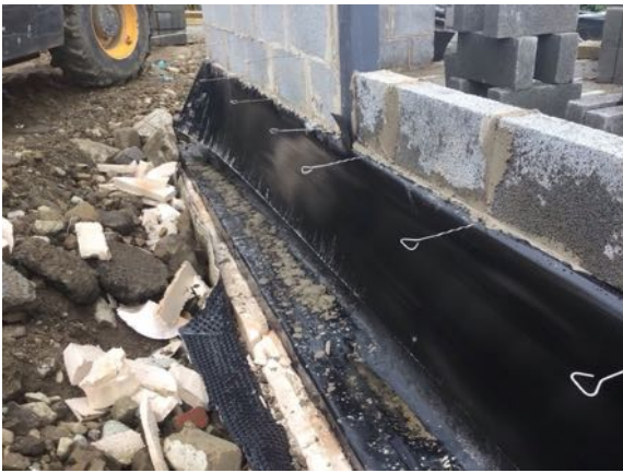
Perimeter retaining wall tanking detail
