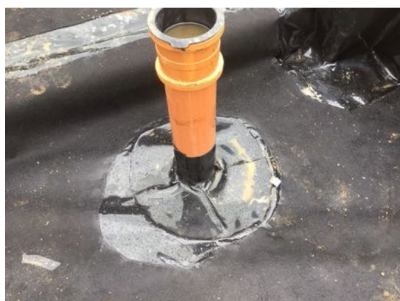
Sealed pipe penetration using Juta Titan tank and heat applied
