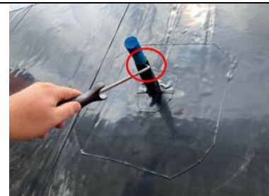
Pick & probe testing upon the sealed 25mm water pipe entry.
