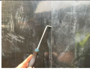
Pick & probe testing to all lapped joints.
