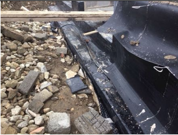
Perimeter retaining wall tanking detail
