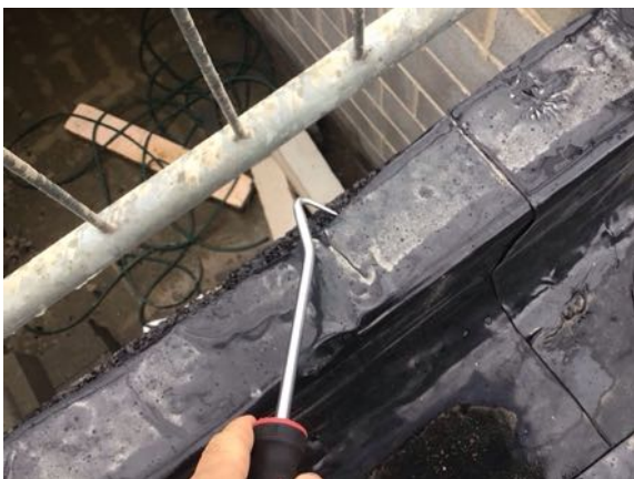
Probe testing seal to pre primed brickwork
