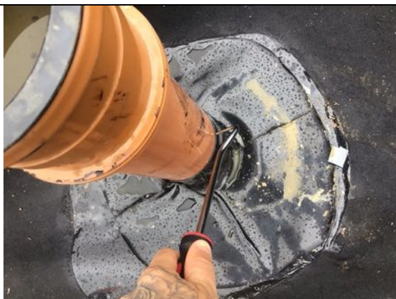
Probe testing pipe penetration
