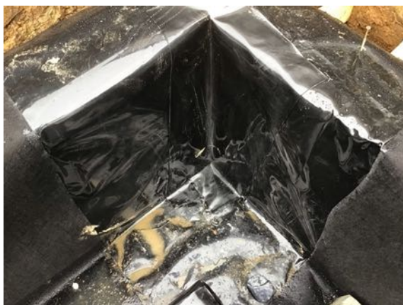
Corner detail sealed using Juta Titan tank and heat applied
