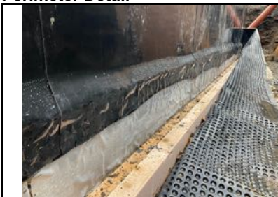
Juta TitanTank membrane sealed to the existing Juta TitanBond gas barrier.
