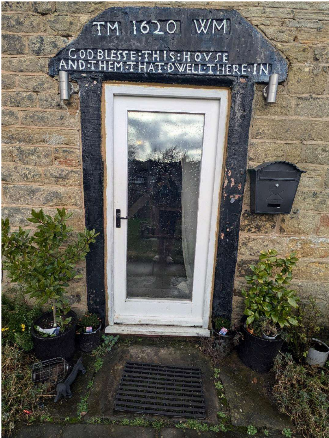
Picture of the temporary replacement door, which we would like to keep
