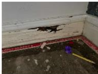
Image 2 A leak was suspected to be occurring from the chimney stack
