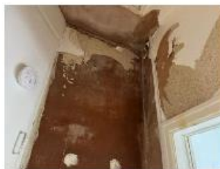
Image 3 A leak was suspected to be occurring from the chimney stack
