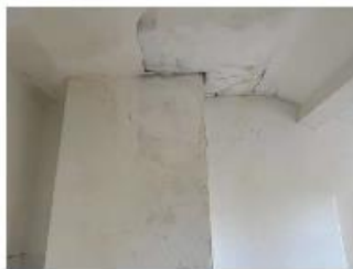
Image 4 Ceilings were damaged by leaks
