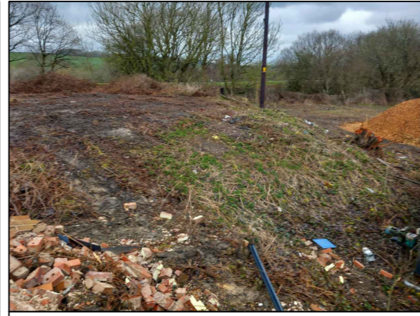
3. Photo of stockpile within east of site, including wooden pole, with area of former infilling and pond beyond to the east.
