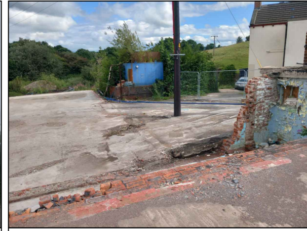
6. View of former AST, prior to demolition and clearance.
