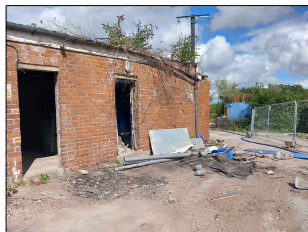
7. View of former sub-station prior to demolition and clearance.
