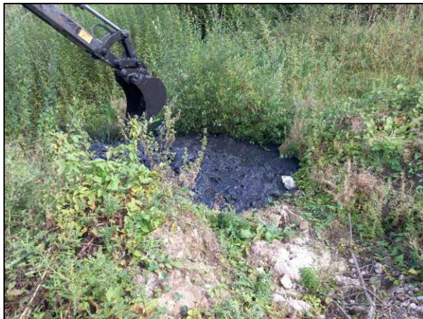
11. View of black saturated pond sediments during trial pitting.
