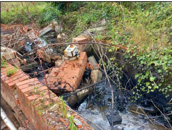
8. Surface water culvert located in southeast, with black oily substance noted.
