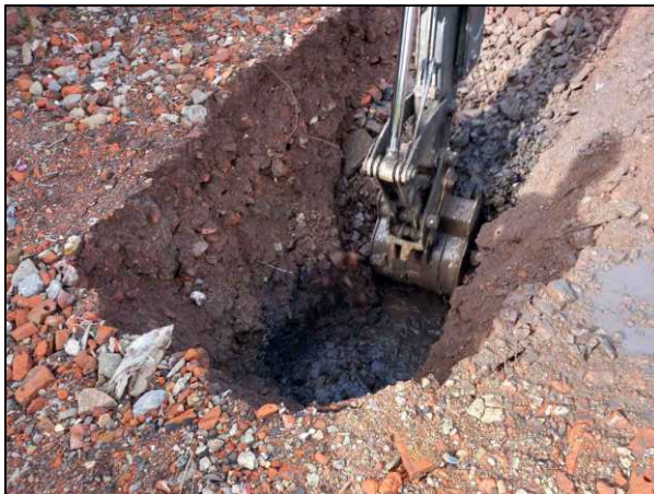
10. Evidence of hydrocarbon staining within backfilled mill pond (trial pit TP218).
