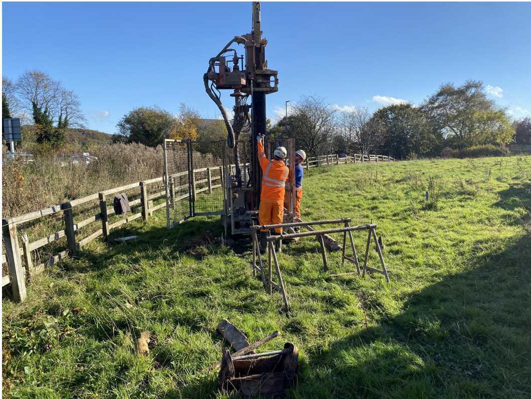
Photograph 1: Rotary drilling rig set up on BH005R(D).
