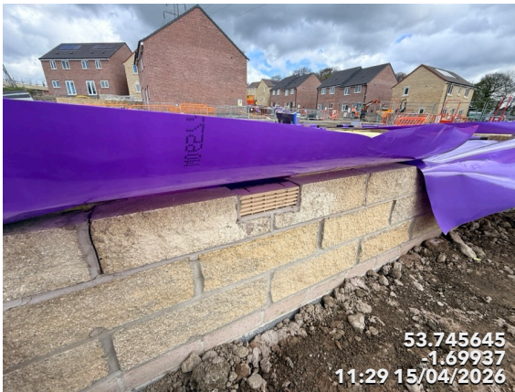
Photo 3 View of air brick
