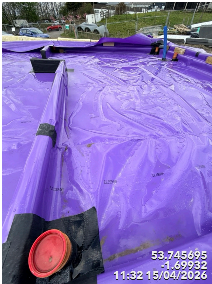
Photo 6 Double heat welds and internal wall element
