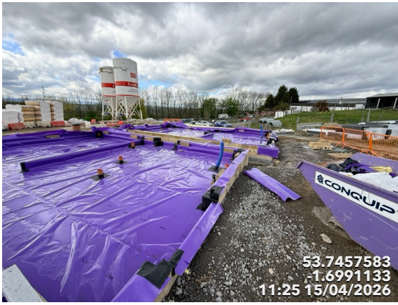
Photo 16 Heat welded joints
