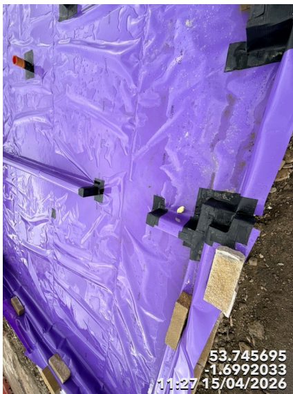
Photo 11 Small hole repair using self adhesive membrane
