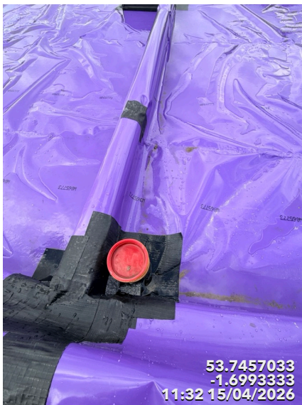
Photo 7 Double corner detail with sealed service entry
