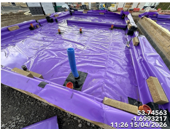
Photo 15 Overview showing total coverage
