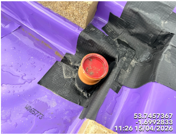
Photo 13 Service entry sealed with self adhesive membrane
