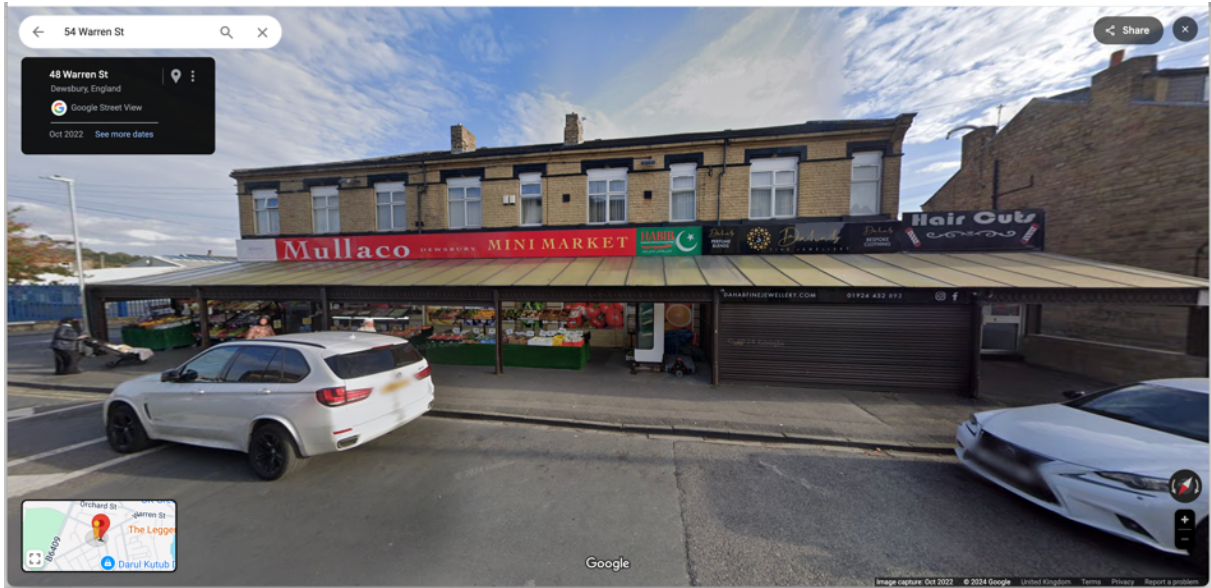
Application Site – Front Elevation 54 Warren Street
