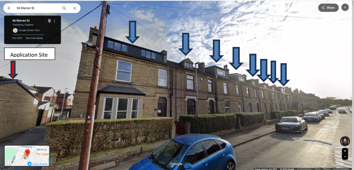
Street View - Warren Street front dormers to adjacent terrace
