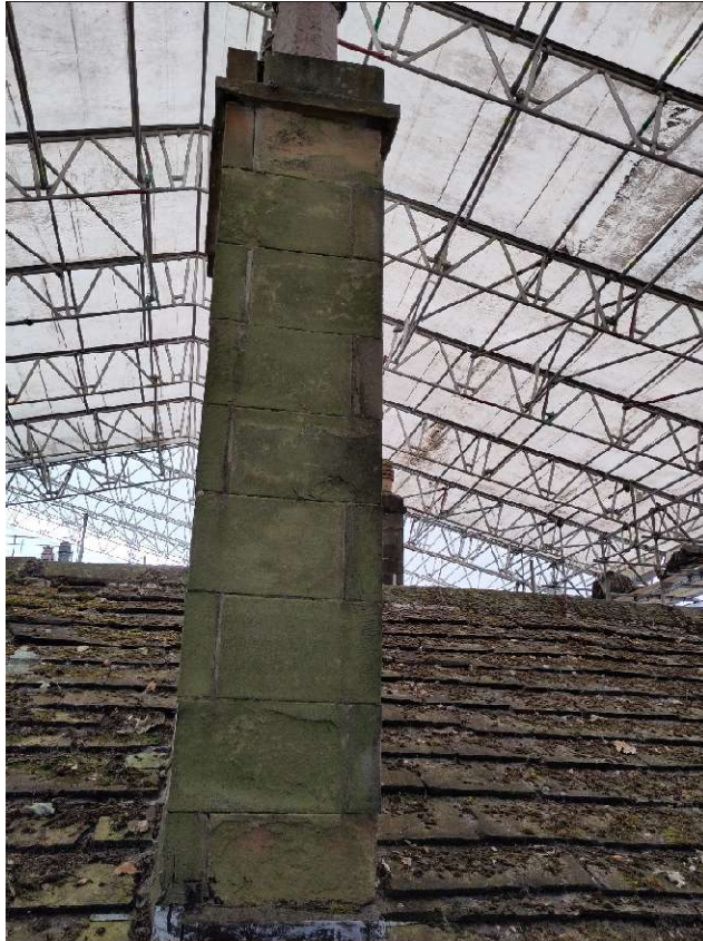
Photo 7 – Stack S2 from West
