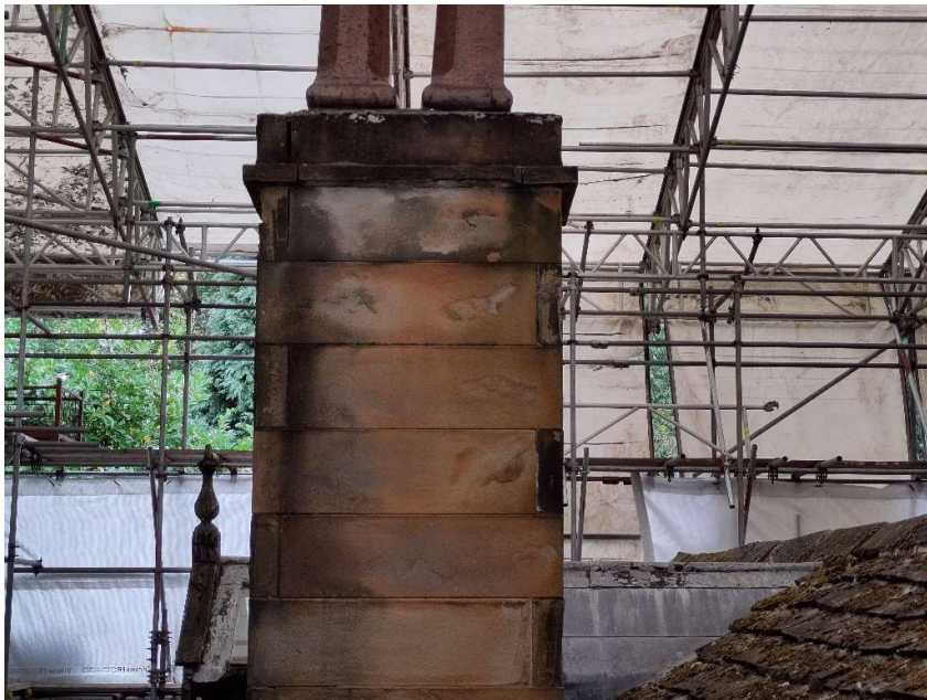
Photo 6 – Stack S2 from South
