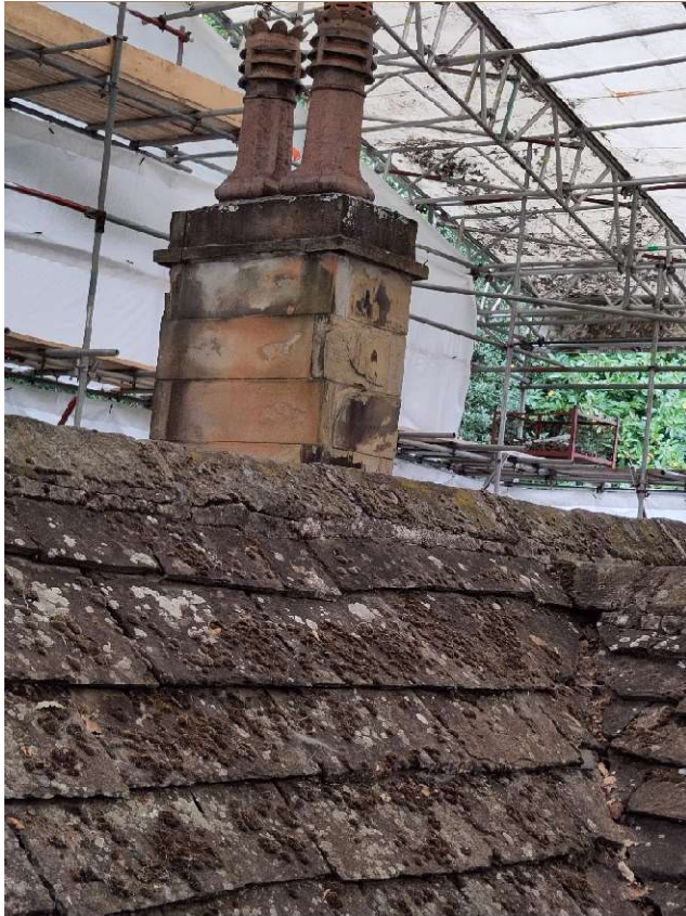
Photo 5 – Stack S2 from South East
