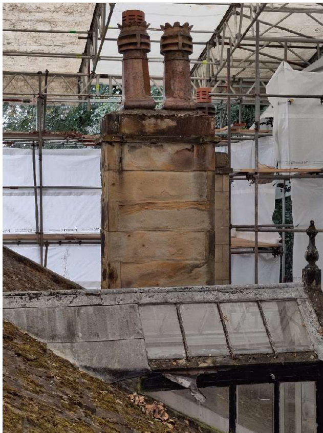
Photo 4 – Stack S2 from North
