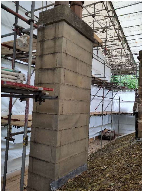
Photo 1 – Stack S1 from South
