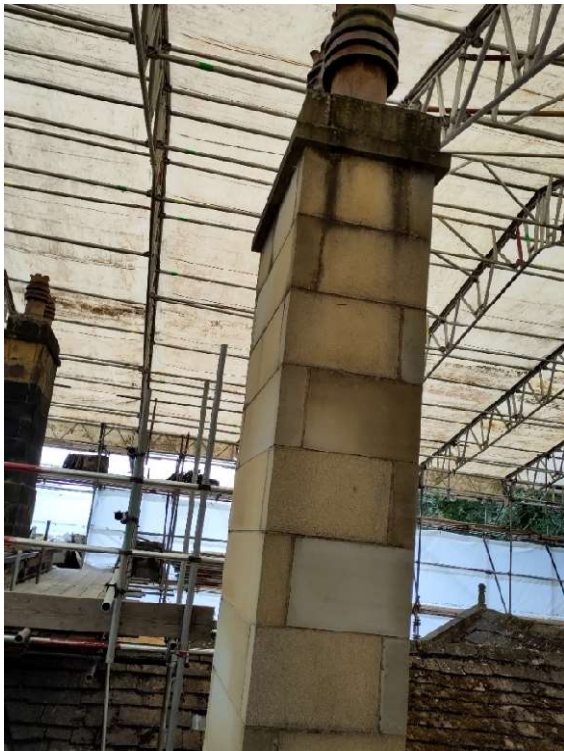
Photo 17 – Stack 4, from North, top section.
