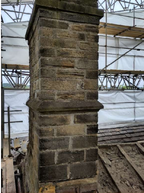
Photo 32 – Stack S9 from West
