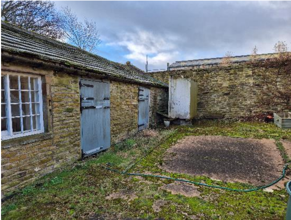
The fuel tank
