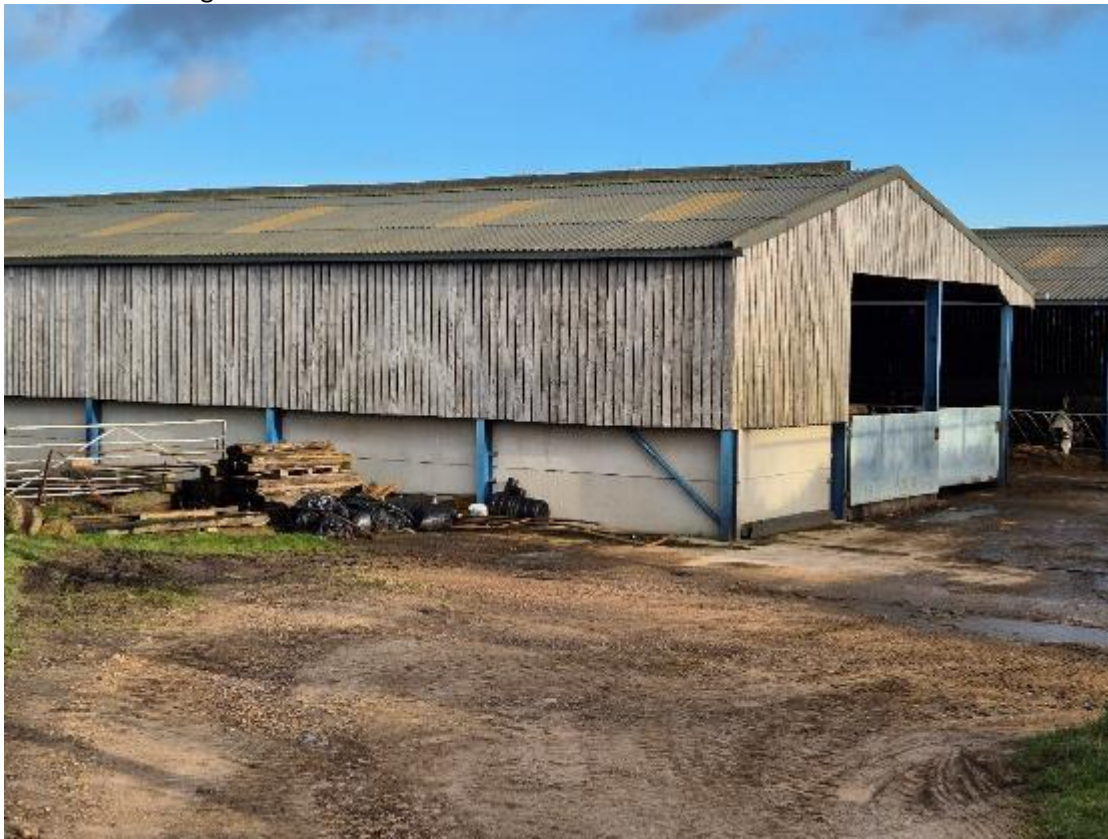
The farm buildings to the west
