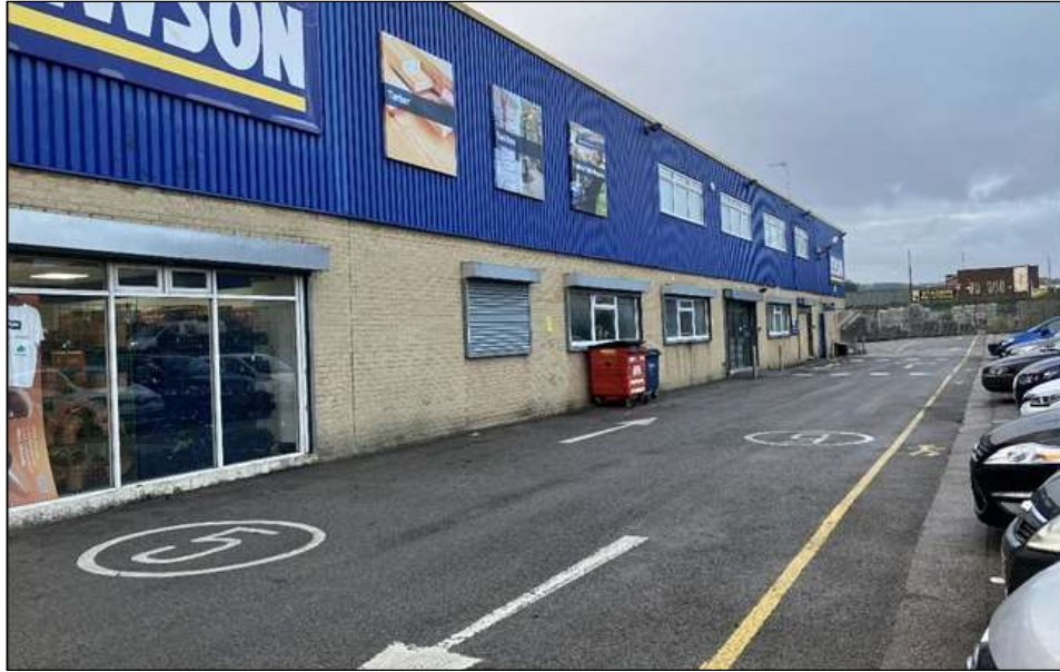
Photograph 1 – Photograph of the warehouse/offices building looking south
