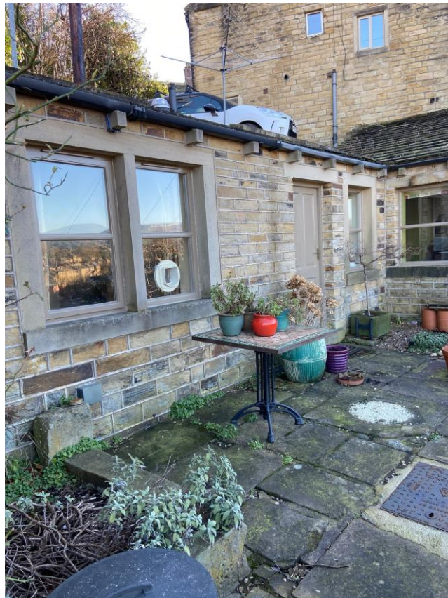
Above: Photos of the existing single storey structure
