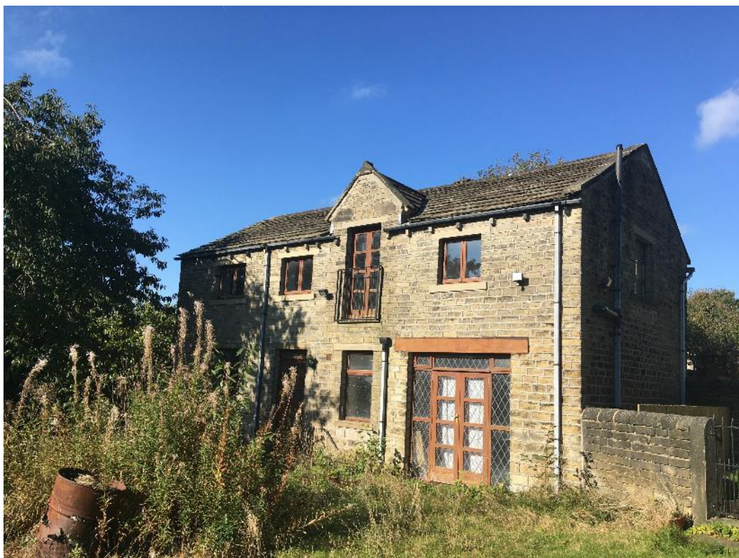
Photo 10. Western-most building, looking west
