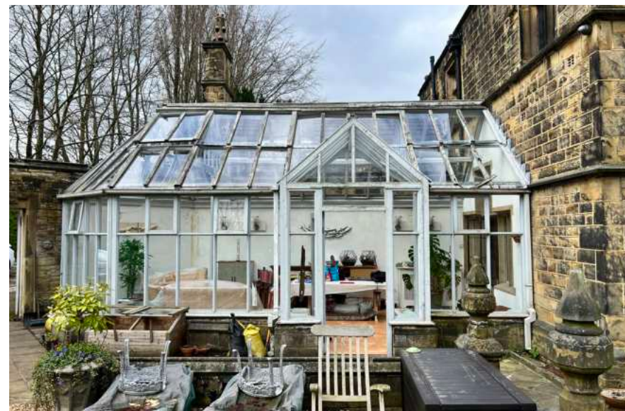
Photograph 2 - Front south elevation of conservatory
