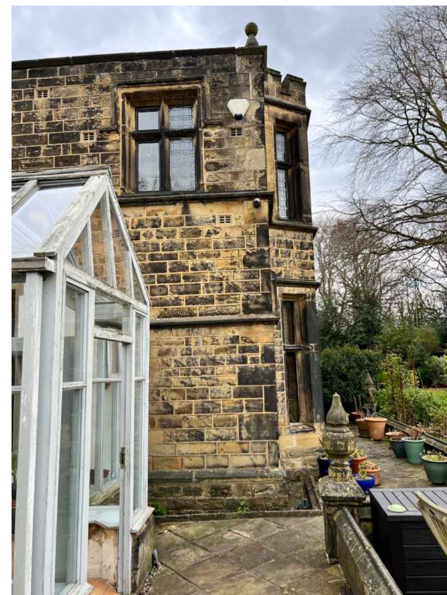
Photograph 12 - Close up view of hall southwest corner
