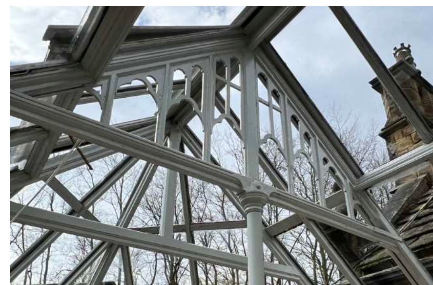
Photograph 6 - Cast iron support to third roof truss
