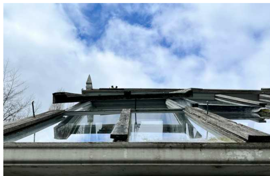
Photograph 4 - Close up view of roof glazing bars
