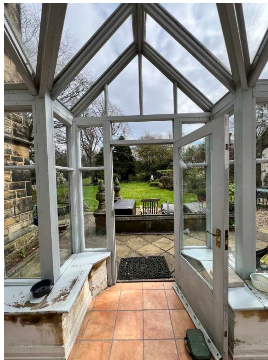
Photograph 11 - View from garden door onto patio
